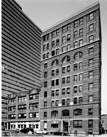
Figure 6. The Matheson Building (1897) in New York, a typical early skeleton building. (HABS/HAER http://memory.loc.gov/ammem/collections/habs_haer/ )
