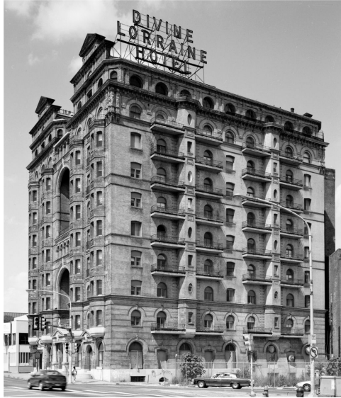
Figure 4. The Divine Lorraine Hotel (1894) in Philadelphia, a typical cage building. (HABS/HAER http://memory.loc.gov/ammem/collections/habs_haer/ )
