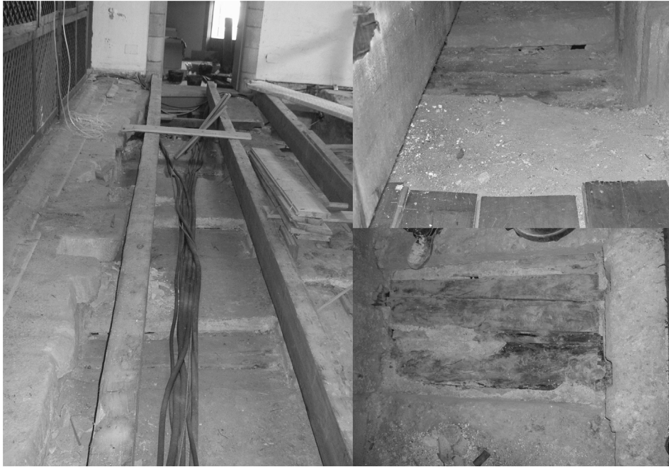
Figure 7. The extrados of the choir vault. Test pits. (Courtesy of R. Saez y A. Parga.)
