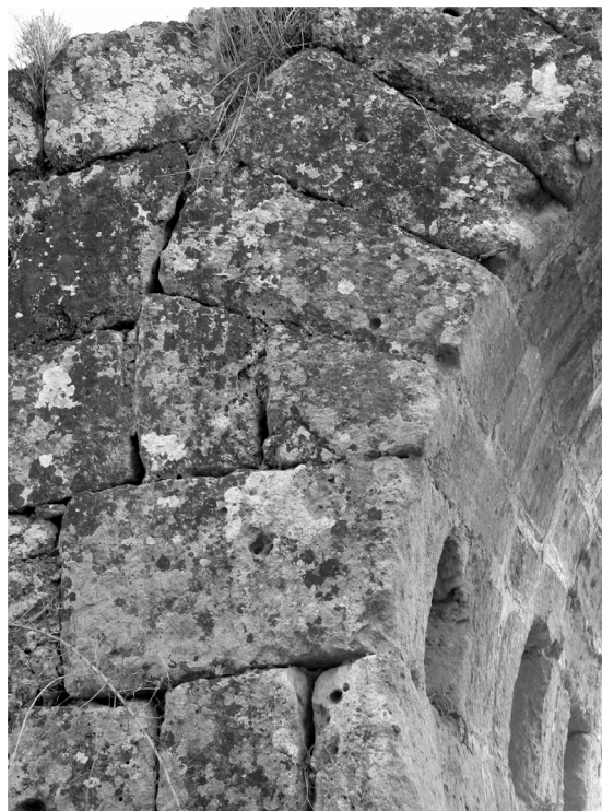
Figure 8. Quebrado Bridge, voussoirs
