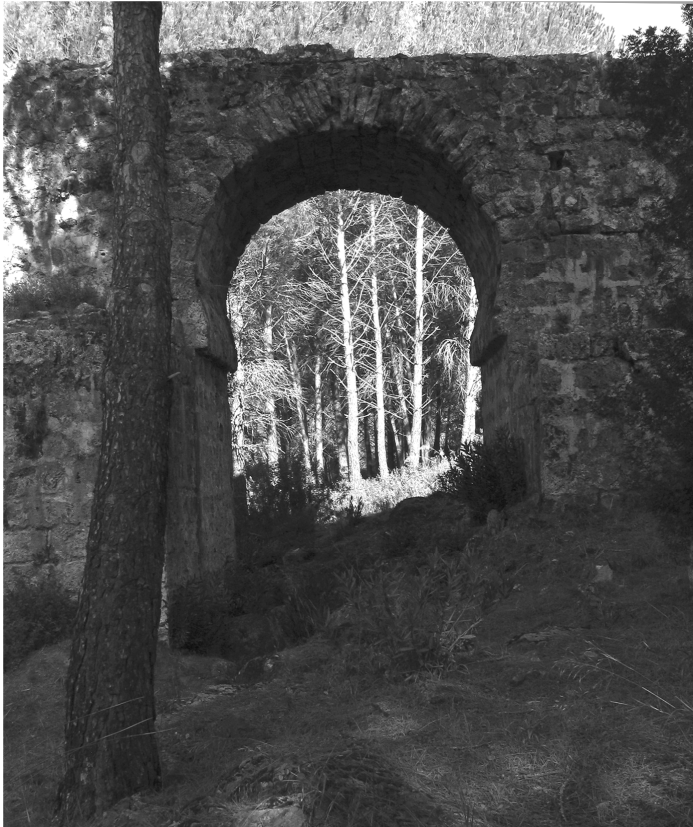
Figure 5. Tejera Bridge, detail.
