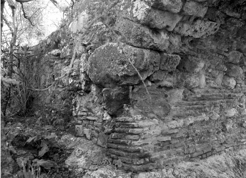
Figure 10. Repairs to Guadalbacar Bridge at the springing of the arch.
