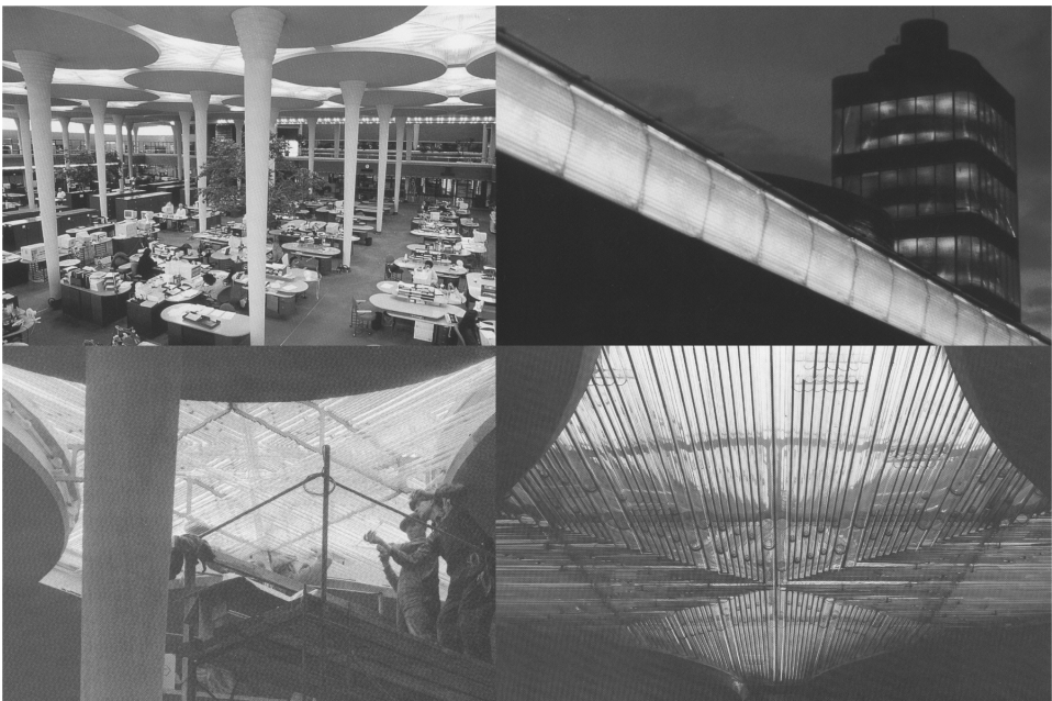
Figure 8. Above: The Great Workroom; Administration Building and Research Tower. (Hertzberg 2004, pp. 56, 59). Below: Pyrex tubes in Great Workroom skylights. (Lipman 2003, pp. 78-80, fig. 79, 82).
