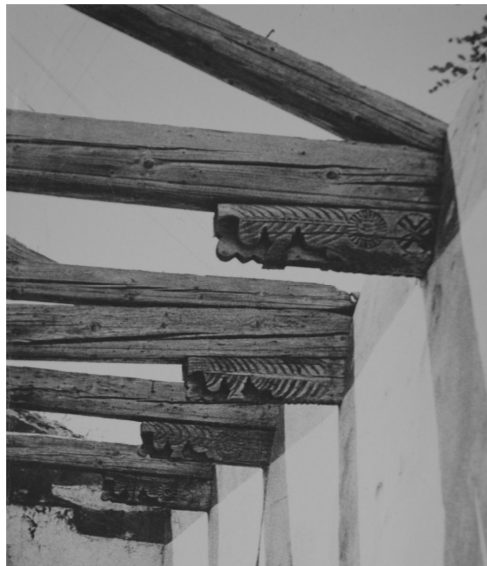
Figure 14. The palm-tree motif on the ancones in St. Michael (Photograph, Archive Soprintendenza of Messina)
