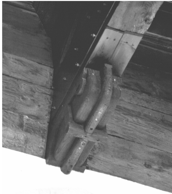
Figure 7. St. Nicholas , Taormina. Roof over the main nave: an ancone with a cross in relief on the bottom section
