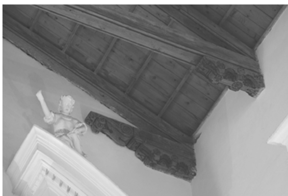
Figure 15. The double ancone in a corner of the roof of St. Catherine's. The difference from a usual ancone (on the right) is very clear
