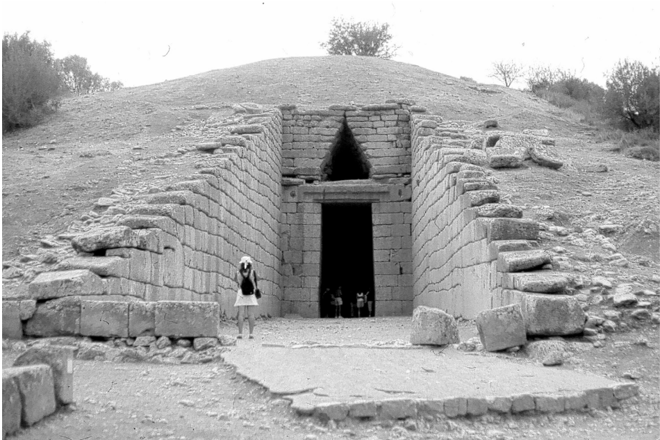
Figure 1. Treasury of Atreus. The dromos , the stomion , and the mound
