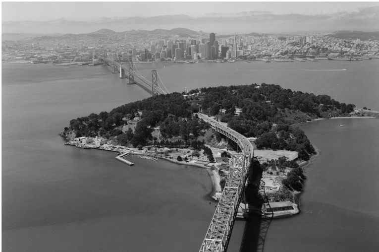
Figure 7. San Francisco-Oakland Bay Bridge, southwest view with Yerba Buena Island, Frank Deras, Jr., photo (Library of Congress, Historic American Engineering Record, HAER CAL,038-SAN FRA,141-81)
