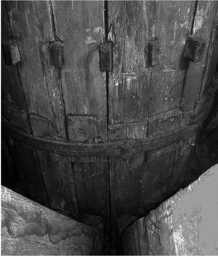
Figure 16. The Woolwich Rotunda’s 24 individual bevelled king posts, strapped together with hinged iron hoops, and fortified against timber shrinkage by wedges and packing pieces. Barrel making might have inspired this arrangement. (Jonathan Clarke).
