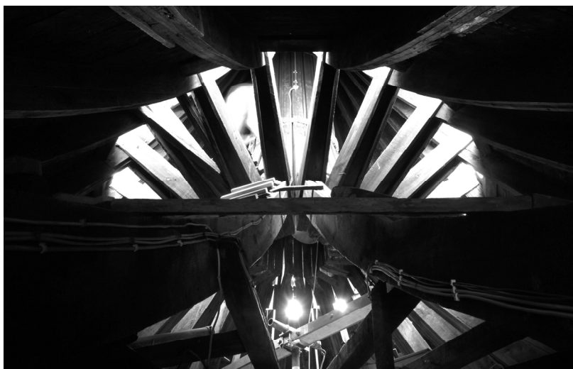
Figure 18. Upwards view towards the apex of the laminated-timber roof over the Music Room, Brighton Pavilion. The inclined members are the array of upper struts, joining the upper and lower chords (Derek Kendall).
