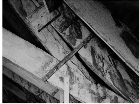
Figure 11. Inverted u-shaped iron stirrup, here fastening the laminated upper chord to two struts (Pat Payne, AA048109).
