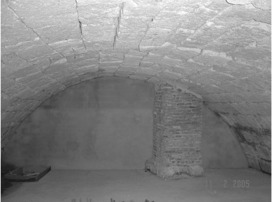
Figure 11. The Costanilla bridge: one of the arches. View from the basement of a newly-made building (Author's photograph)
