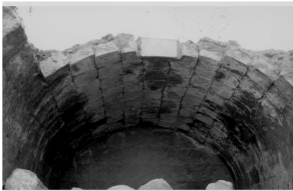
Figure 3. Type of haunches of a barrel vault.
