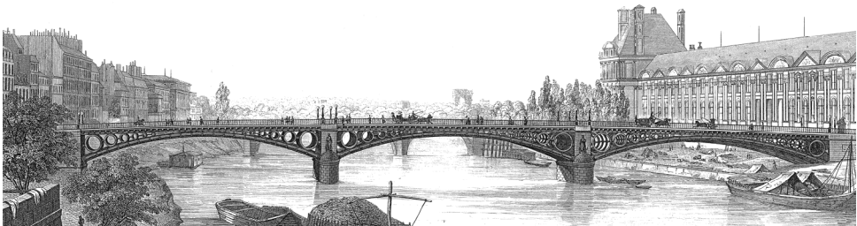
Figure 1. Carrousel Bridge, 1834. (Polonceau 1839, lam. I)
