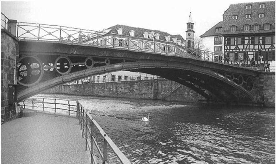
Figure 3. Saint Thomas Bridge, 1841. (Fernández Troyano 1999, p. 331)
