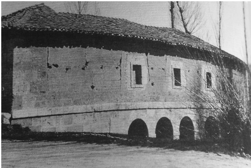
Figure 2. Eighteenth century typical Mill with rammed earth walls (Helguera 1992, p. 36).
