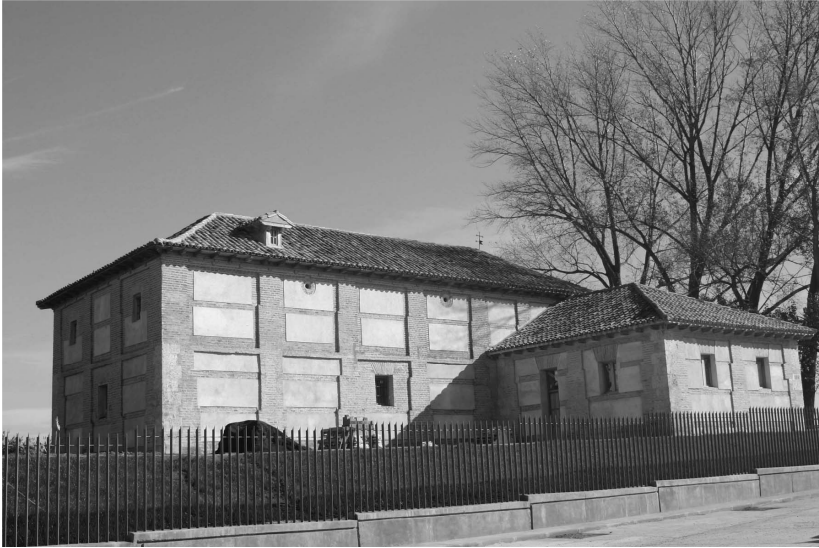
Figure 13. Casa del Rey , built with bricks and rammed earth.
