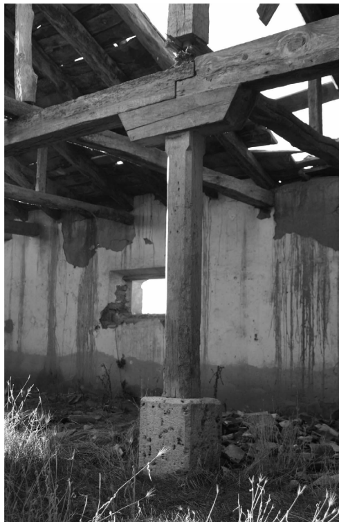
Figure 4. Current wooden and adobe structure in the Canal's buildings
