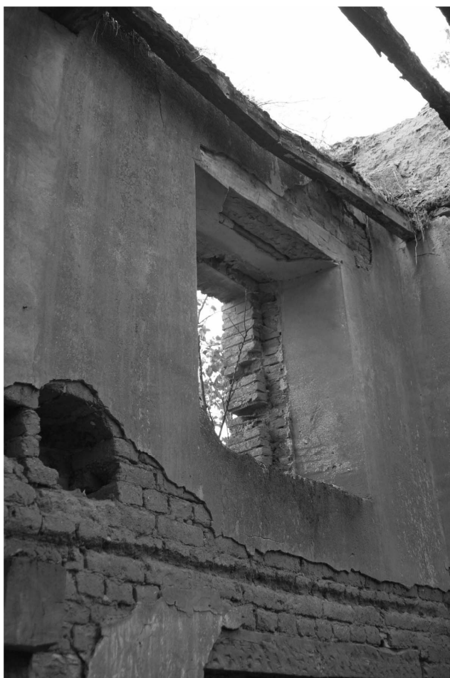
Figure 5. Adobes in the inside of the brick walls in a view of Batan del Rey .
