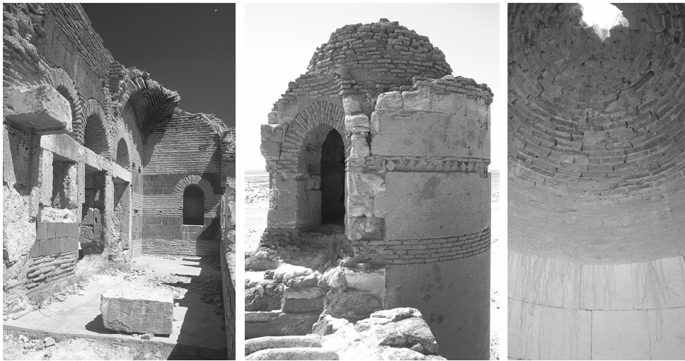
Figure 6. Mixed Brick & Stone masonry of Byzantine tradition. a: Qasr Ibn Wardan, Justinianic pretorium using basalt, limestone & brick; Qasr al Hayr as-Sharqi. Domes on hollow towers, b: exterior; c: interior.
