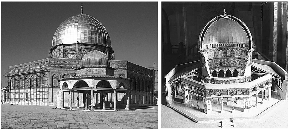
Figure 13. Wooden Domes. Jerusalem. a: Dome of the Rock & Dome of the chain; b: Dome of the Rock, section (model from the David’s Citadel Museum).
