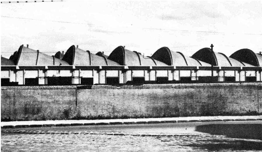
Figure 2. Railway workshop in Bagneaux, France, designed by Freyssinet. Conoidal Vault reinforced by stiffening beams in the upper side (Fernández 1978, fig.72)
