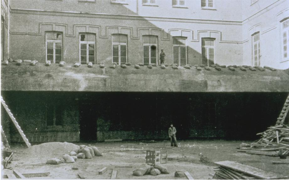
Figure 8. View of the shell built without the stiffening beam after the load test was finished with satisfactory results (AET, file number 275).
