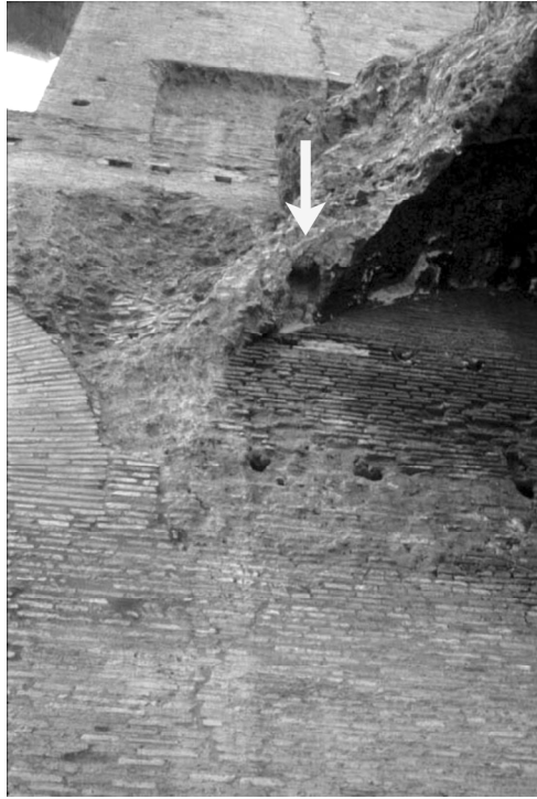
Figure 7. Porch, north end. Remains of a well-preserved terracotta tube at the spring of a cross vault placed perpendicularly to the exterior limit of the upper wall.
