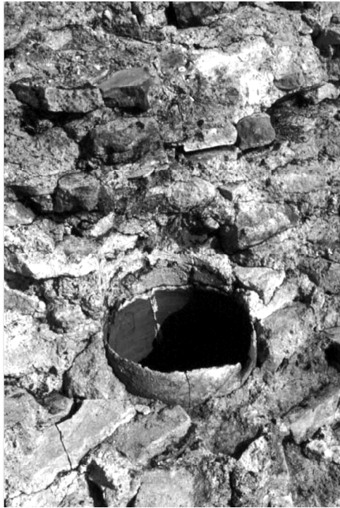
Figure 10. Remains of a series of vertical terracotta tubes with a 25 centimetre diameter and 250 centimetre height buried in the remains of the vault. Concrete above the ribbed sections of the vault was made lighter by the use of tuffo giallo and grey pumice.
