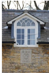
23 and 24 Main Street, Blatherwycke [Figure 19] features intricate glazing bars consistent with later date. 44
