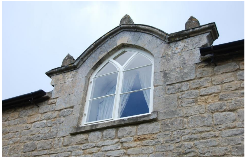
Figure 17 – Dormer window with Gothick pointed arch and 'Y' shaped timber mullion window.
