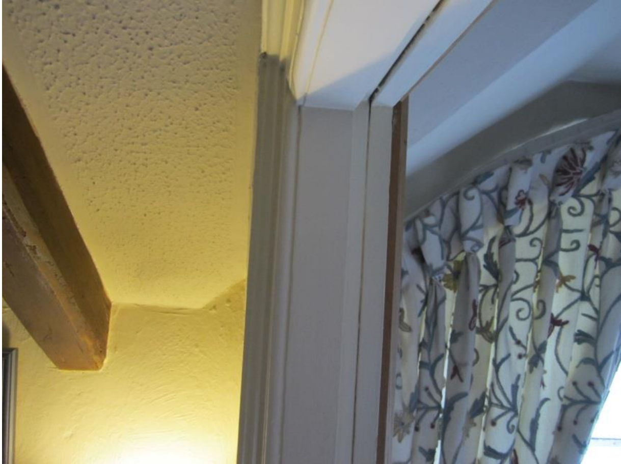
Figure 36 – Wall interrupts intersection of ceiling with dormer.
