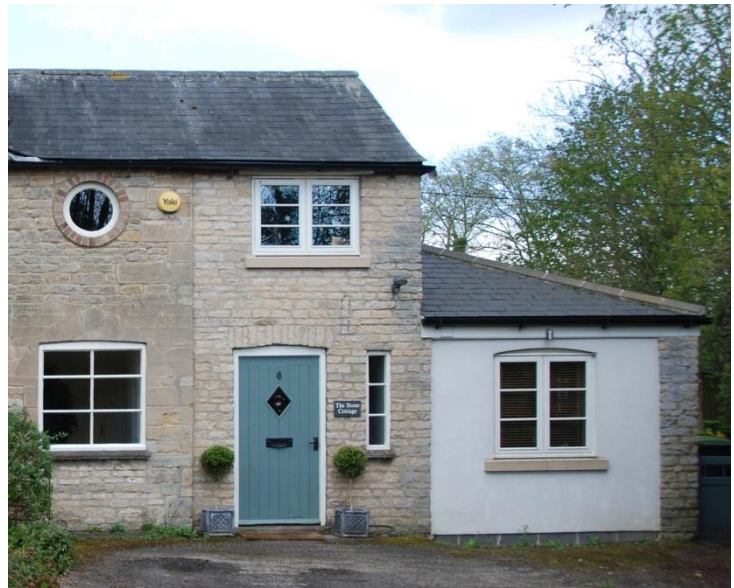
Figure 24 – P6 extension with Welsh slate roof and rendered walls
