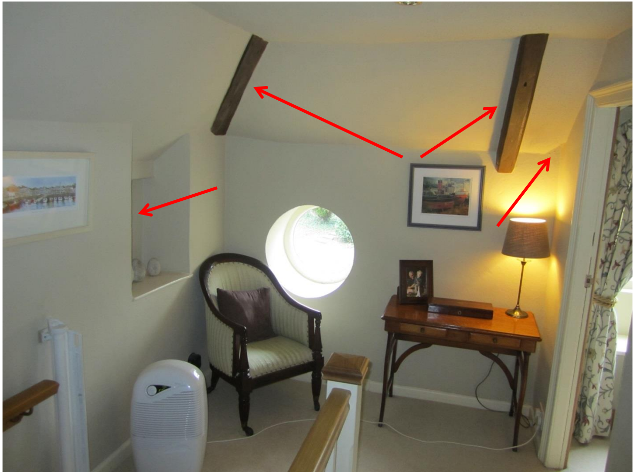
Figure 35 – First floor landing at the top of the stairs. Common and hip rafters exposed with chamfered edges.
