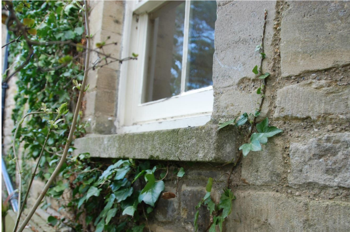
Figure 29 – Window sill for boxed sash window in northeast elevation.
