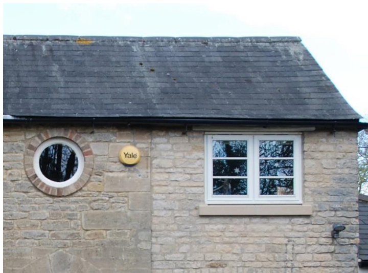
Figure 23 – Round ‘bullseye’ window and new timber casement.
