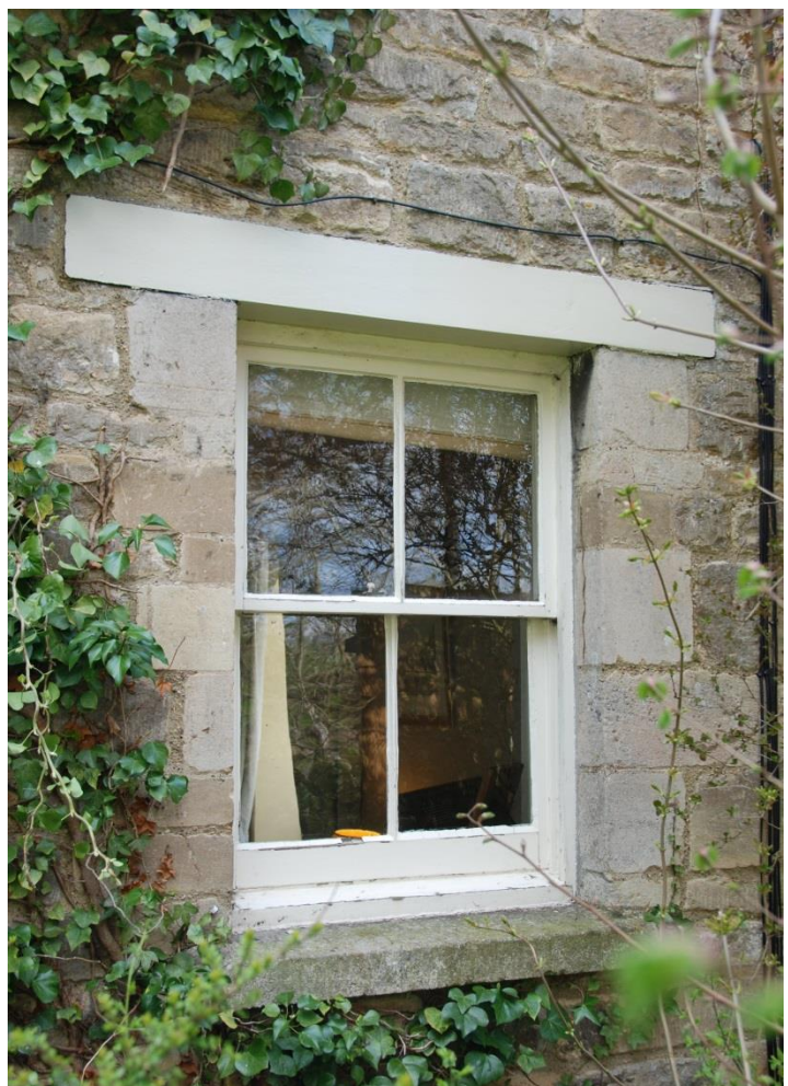
Figure 28 – Fixed casement timber window in northeast elevation.
