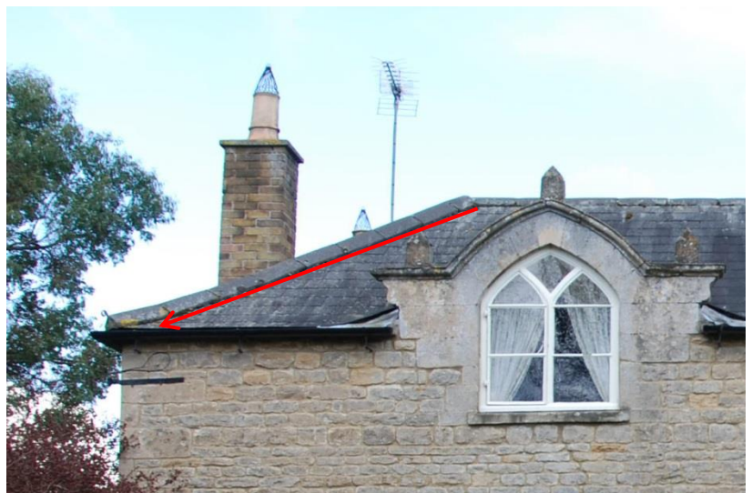
Figure 16 – Hipped roof with sprocketed rafter ends exaggerated by the straight red line
