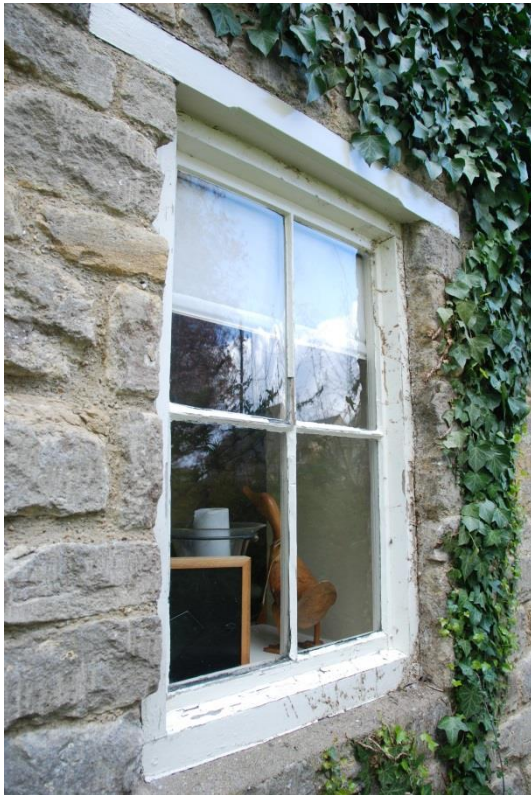
Figure 27 – Fixed casement timber window in northeast elevation.
