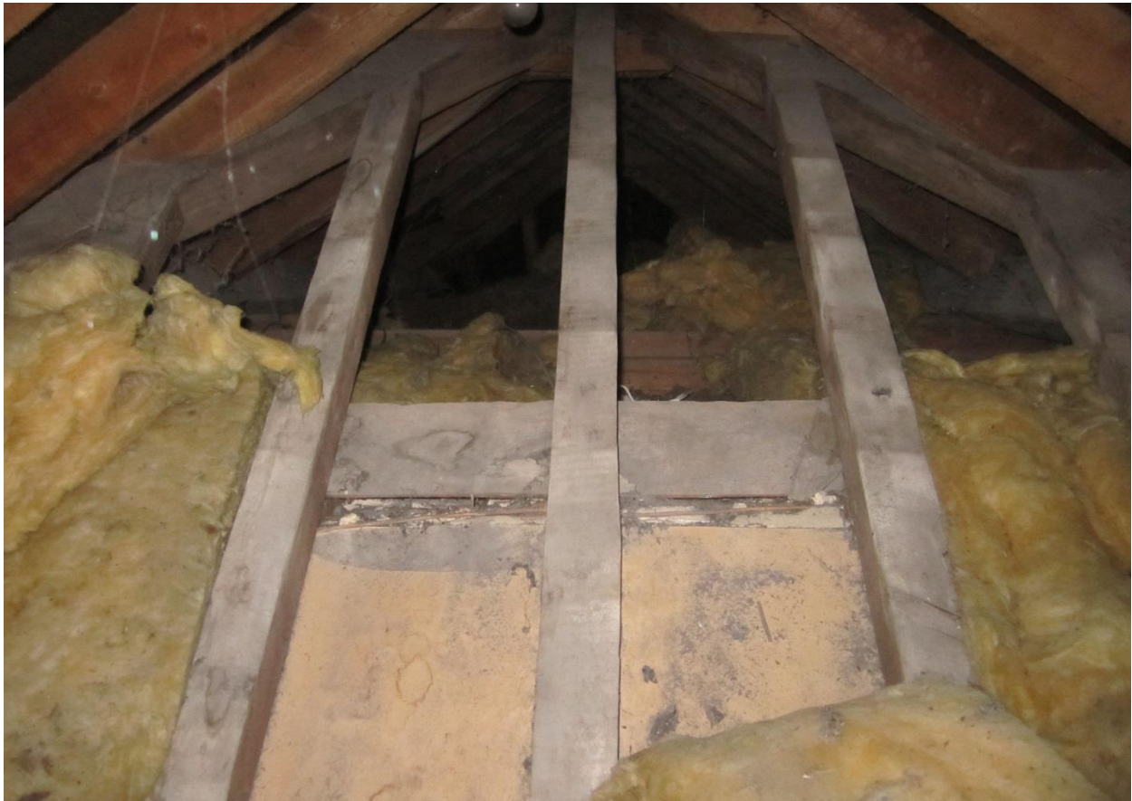
Figure 34 – P1 roof structure evident from attic space. New timbers have been laid over the existing structure.
