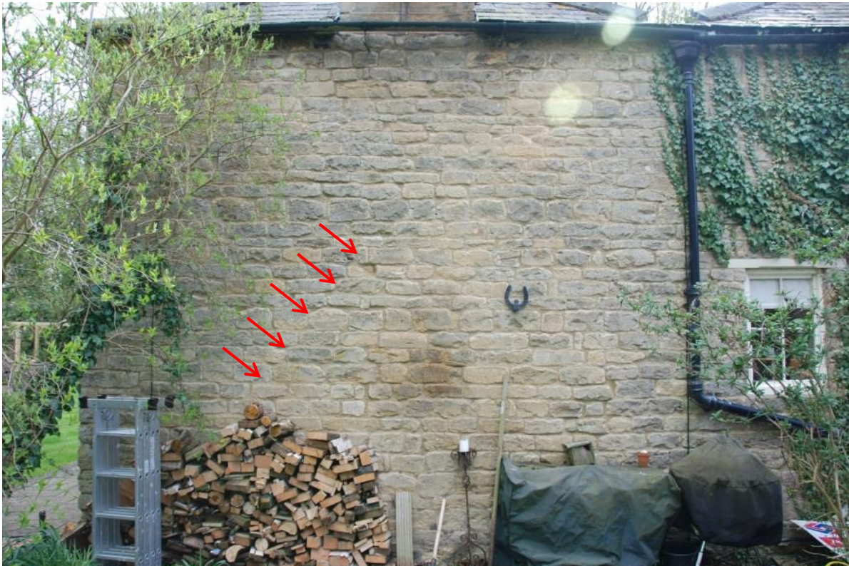
Figure 26 – Forensic scarring from earlier extension, highlighted by red arrows.
