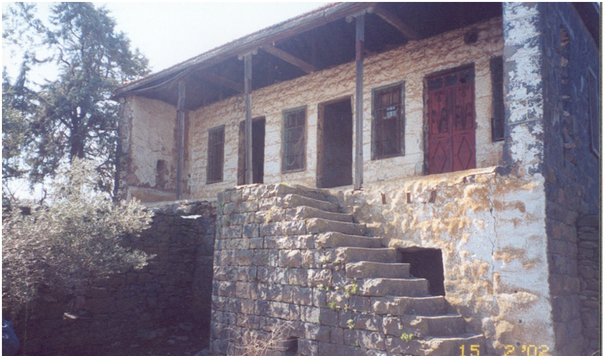
Figure 7. Photos of the ruins of Circassian houses in Bereka, the only remaining Circassian village in the Golan Heights of Syria [Source: Private Files of Architect Amjad Alkoud]
