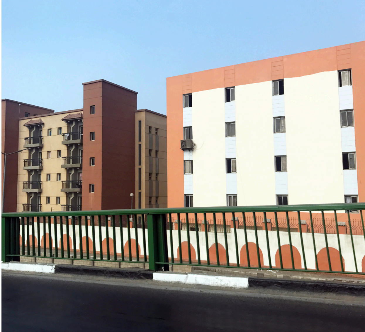
Figure 3. Maintenance extending to adjacent buildings. Authors own
