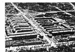
Figure 6. Cells II and I: Aerial view showing buildings under construction.
