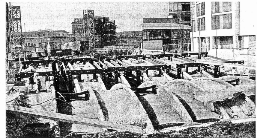
Figure 7. A general view of the structure from the north-east after the removal of the road filling from alternate bays. (English Heritage).
