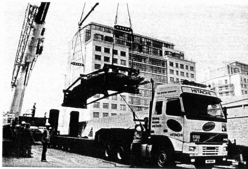
Figure 15. Lifting out the first pair of girders, 31 March 2004. (Malcolm Tucker)
