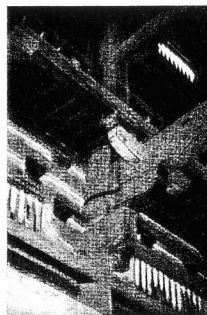
Figure 12 C. Column between corners ( chanzhu bianzao ): library of Longxing Temple, 12 th century, Zhengding, Hebei.
