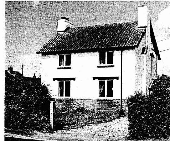
Figure 12. DSIR cottage in rammed chalk-cement at Amesbury, 1920.
