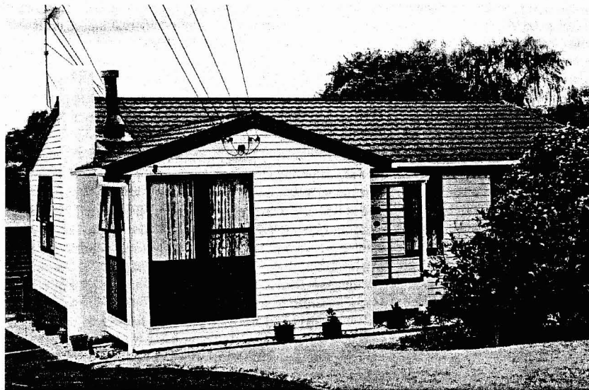
Figure 3. A new roof, a wood burner and aluminium windows. An upgraded pre-cut house.
