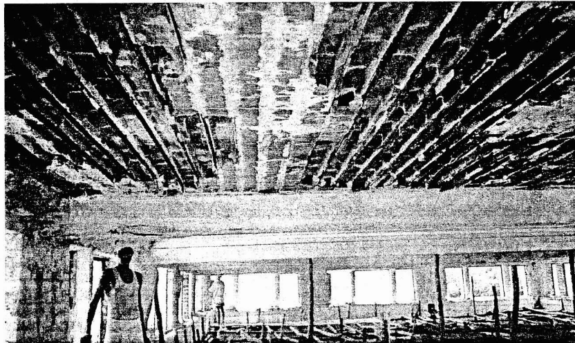
Figure 12. Underside of the Kleine floor system at Freemason’s Hall, Madras.
