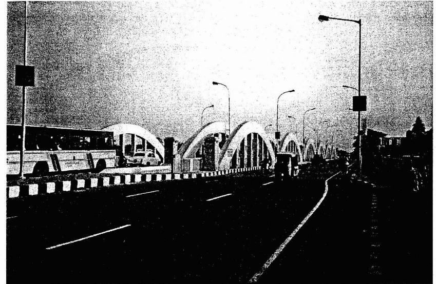
Figure 7. Napier Bridge Madras.
