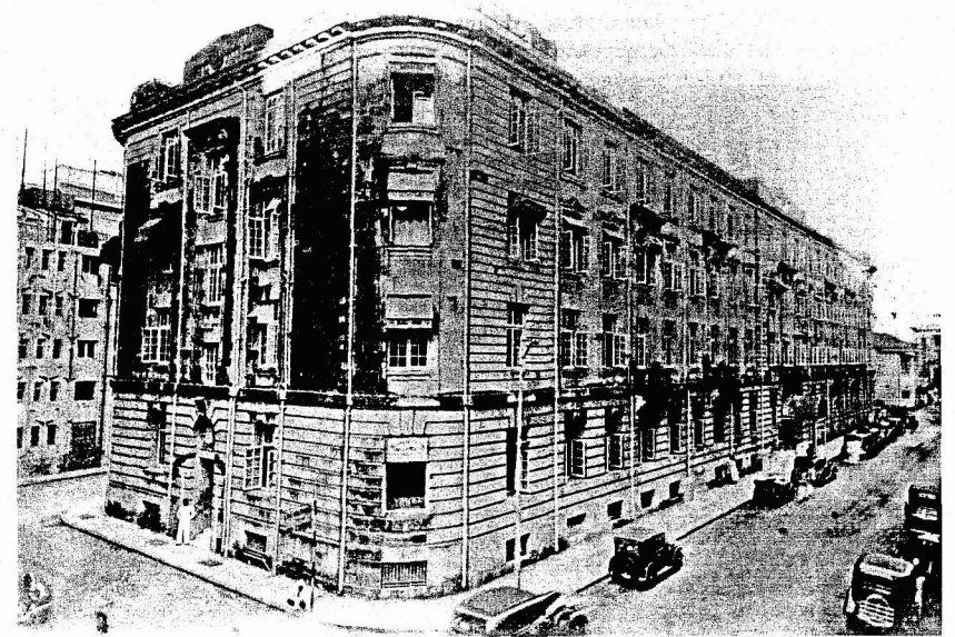
Figure 11. Bombay House, Nami Mody Street, Bombay.
