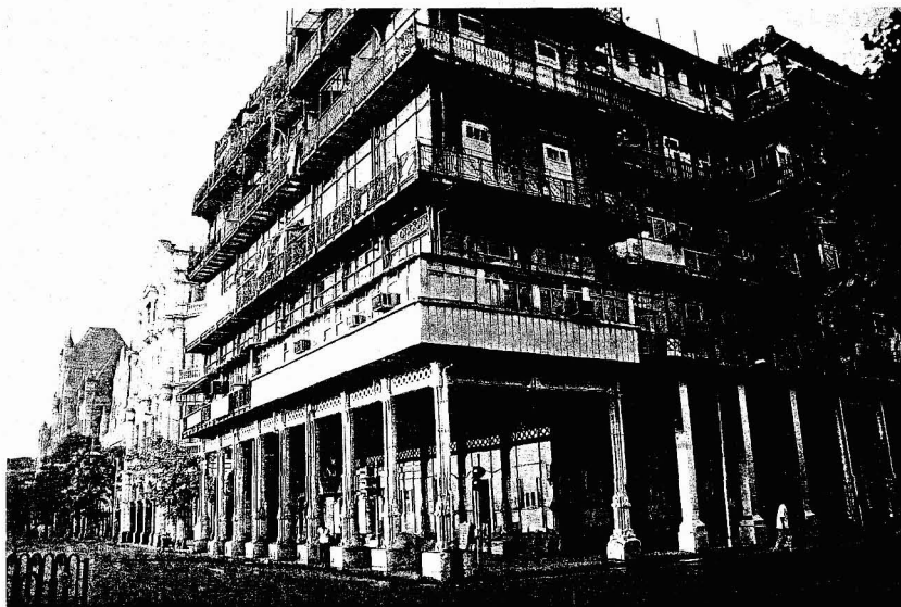
Figure 1. The former Watson's Esplanade Hotel (1867-71), now called Esplanade Mansion (Jonathan Clarke).
