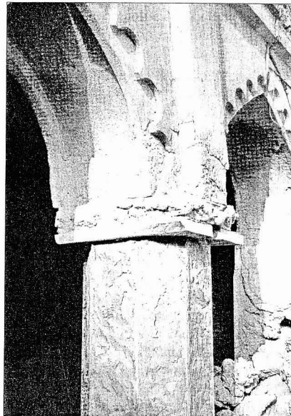
Fig. 8 Arch construction showing permanent formwork, with decorative rendering of extrados
