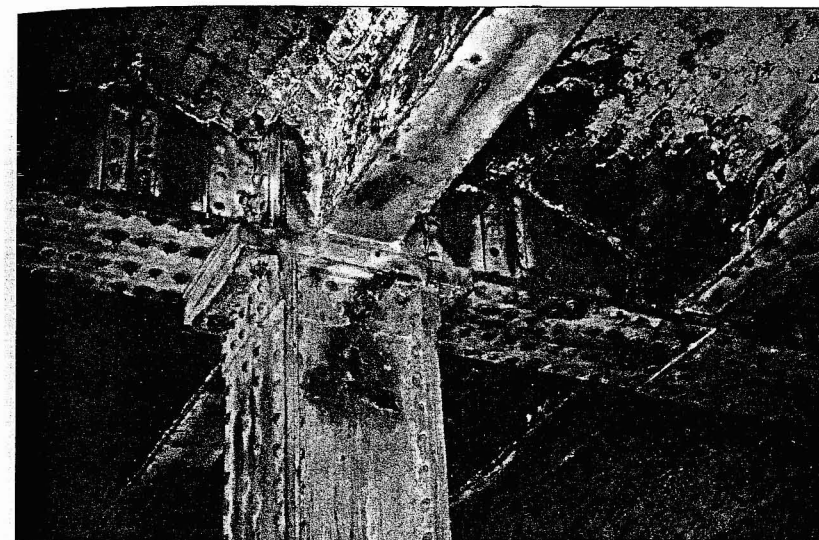
Fig. 4 The Great Northern Warehouse, Manchester (1895-99). Compound steel stanchion supporting steel girders, showing stanchion break at floor level and cast iron seating for floor girder (Alastair Jackson).
