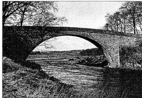
Fig. 5 Keig Bridge, Aberdeenshire, 1817 (Thomas Day)
