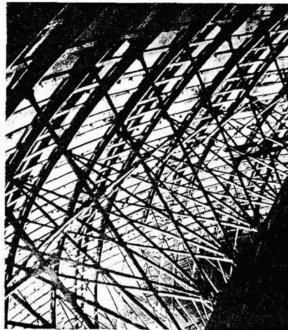
Fig. 24 St. Isaac's Cathedral: interior view of the dome, between the conical dome and the outer spherical dome (photograph courtesy of Professor Rainer Graefe).
