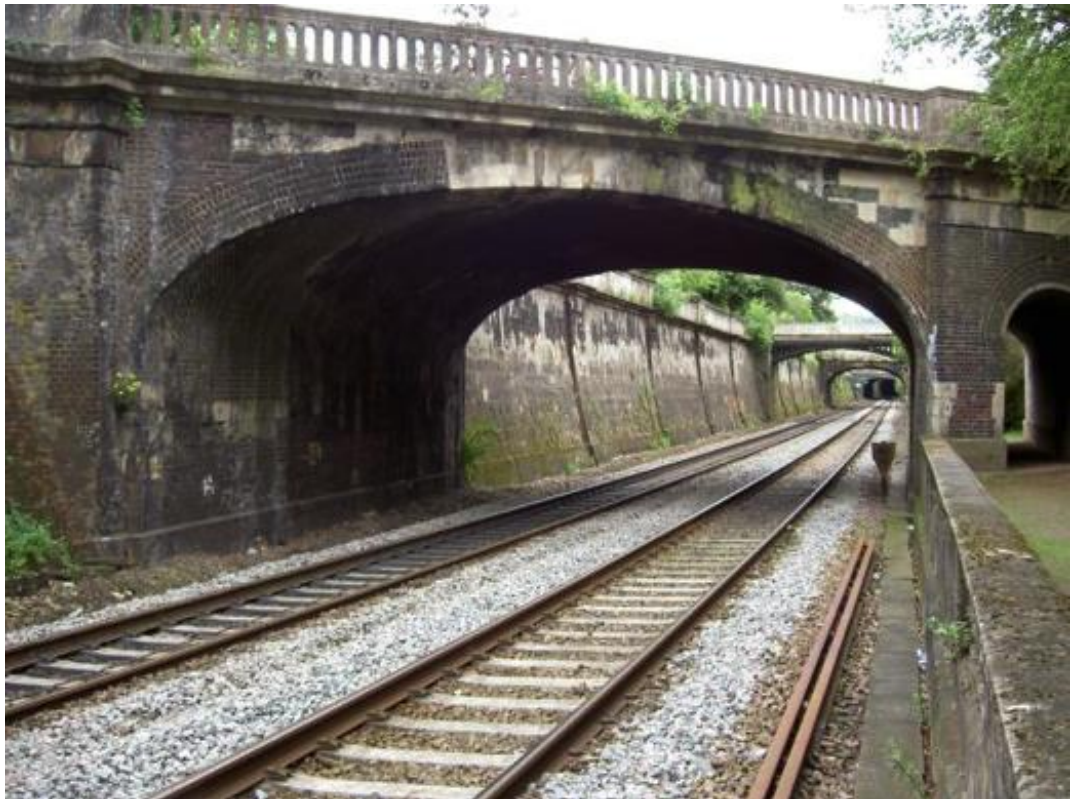
Fig. 2 The Great Western Line in Sydney Gardens (Alan Baxter & Associates LLP)
