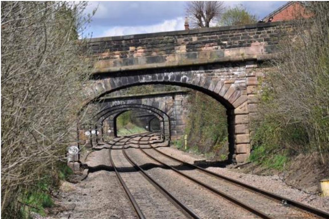
Fig. 4. The North Midland Railway in Belper (Alan Baxter & Associates LLP)
