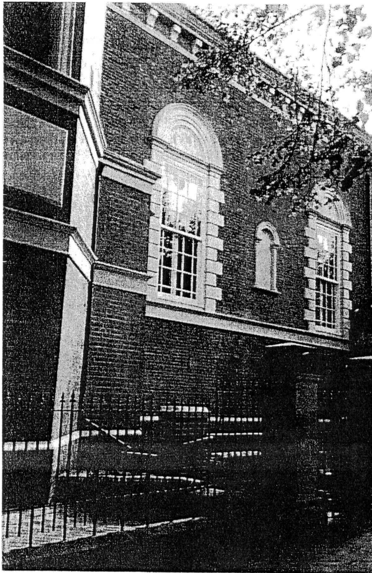
Fig. 4 St Austin's church, Wakefield: windows showing small circular lights at the top.
