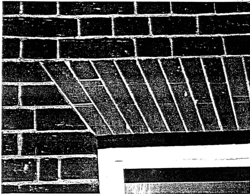
Fig. 1 Skewback, angle of 54°, Aldeburgh, Suffolk
