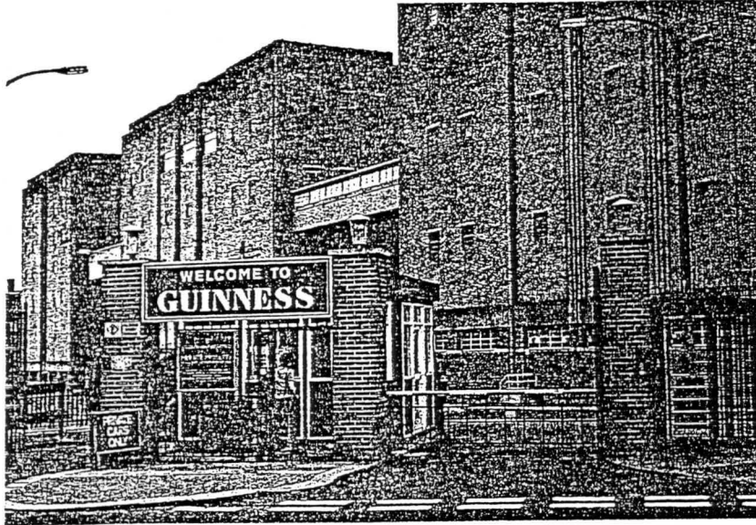
Fig. 6 One of the largest new industrial buildings of the 1930s was the Guinness Brewery at Park Royal in west London, designed to employ 4000 workers. Particular brickwork features are the substantial massing, the vertical ribs and the parapet in soldier courses. The architect was Sir Giles Gilbert Scott.
