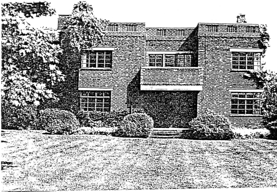
Fig. 4 House of modern design in Stratford-upon-Avon built for a local industrialist, Barney Joseph. The architect was H.W. Simister of Birmingham. The main brickwork is in Flemish Garden Wall bond but in the parapet Flemish bond is used.
