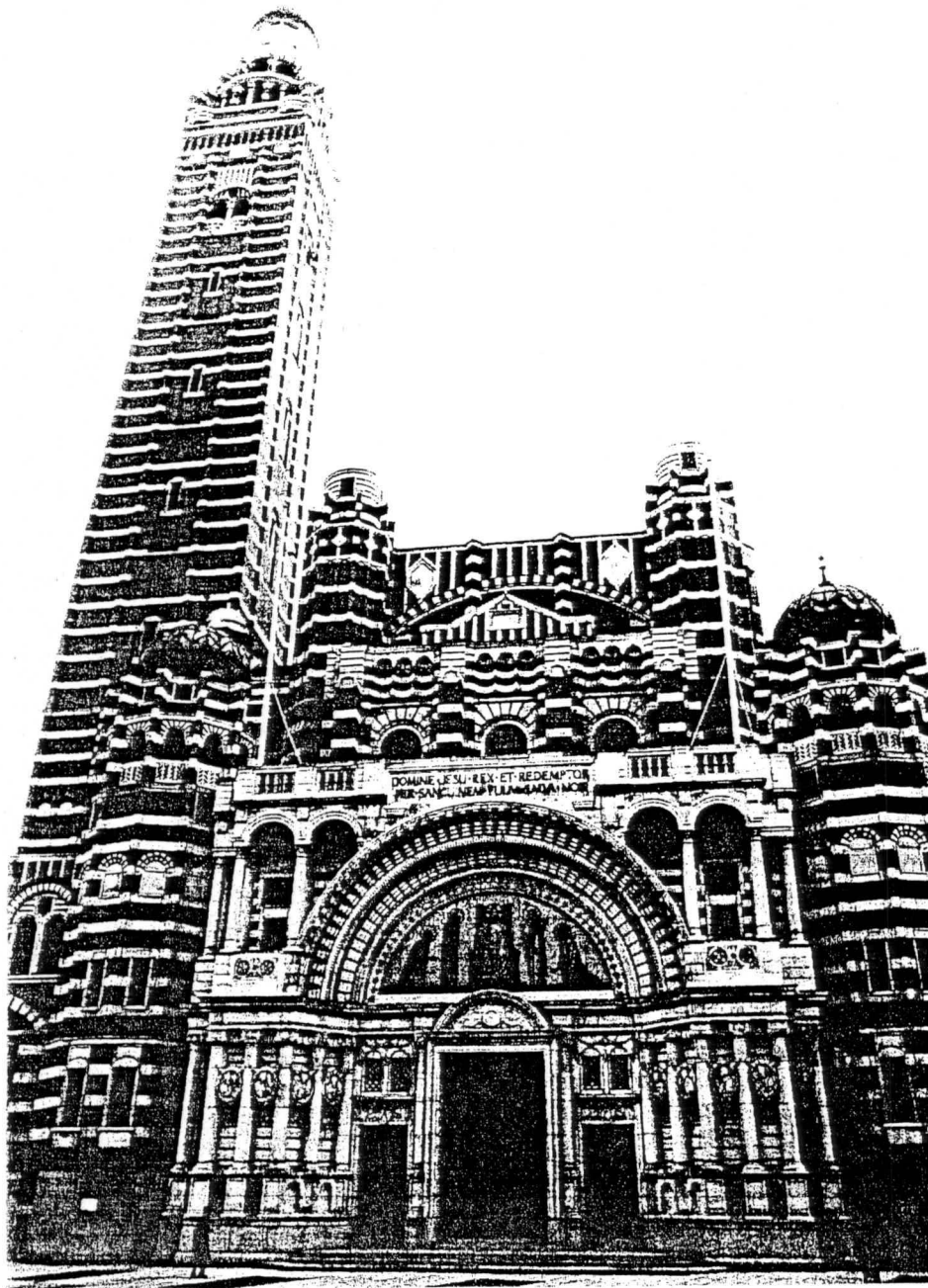
Fig. 3 Westminster Cathedral, designed by J.F. Bentley, in red brick and bands of stone: a tour-de-force of load-bearing brick.
