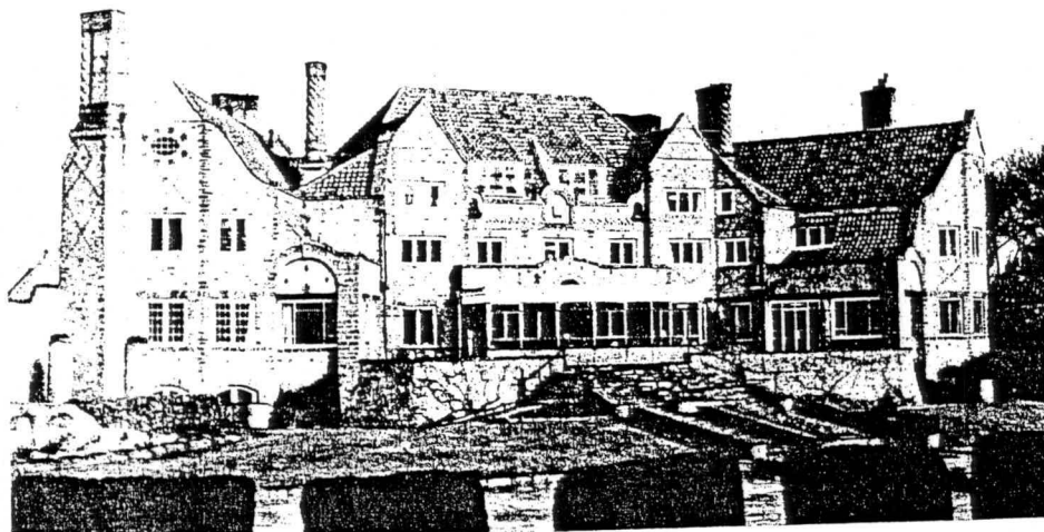
Fig. 2 An architect who used locally-produced materials was E.S. Prior. In the last of his "butterfly houses" at Home Place, Holt, Norfolk, the materials literally came out of the ground on which the house was built. Brickearth was dug from the sunken garden in front of the house. The bricks are used as accents in the flintwork, from flints picked up in the vicinity. The house has been a convalescent home for many years and has been altered both internally and externally.
