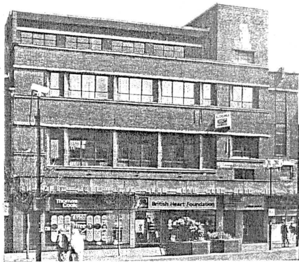
Fig. 9 Former Gas Company showrooms, Luton
