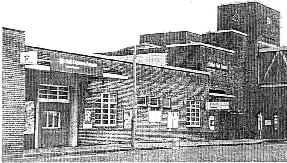
Fig. 7 Luton (formerly Luton Midland Road) Railway Station
