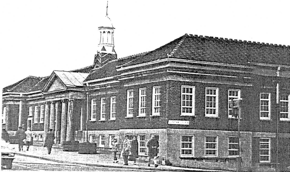
Fig. 4 Police Station and Law Courts, Luton (demolished)
