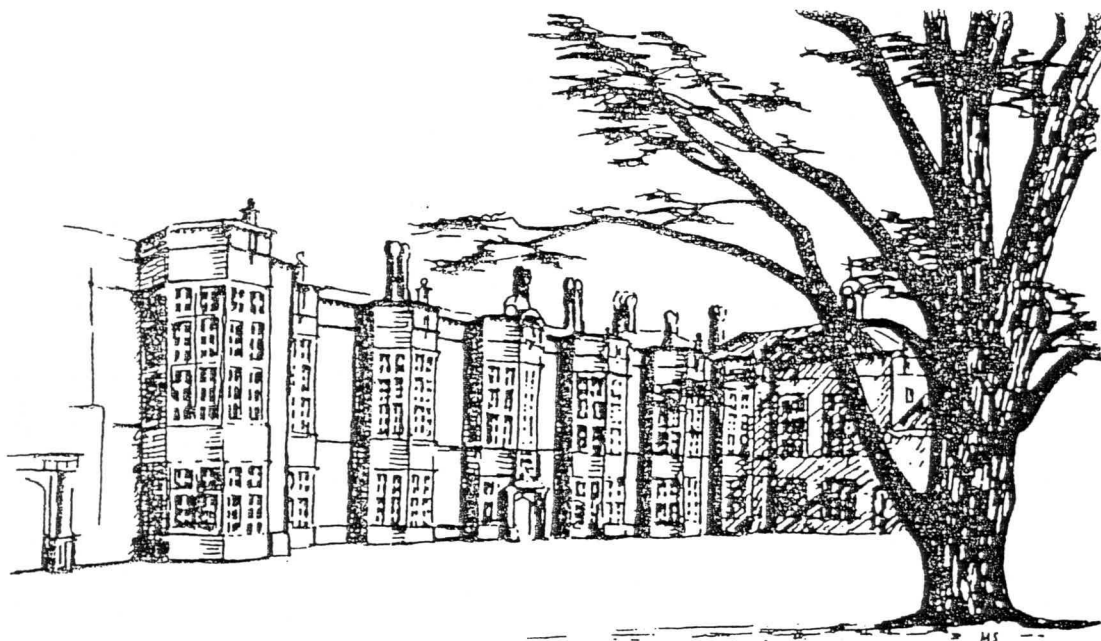
Fig. 2 New Hall, Boreham, Essex. Six of the seven bows of the 1573 front to the 1517 of the north range of Henry VIII's quadrangular palace. The seventh bow is hidden behind the 1920s range on the left.
