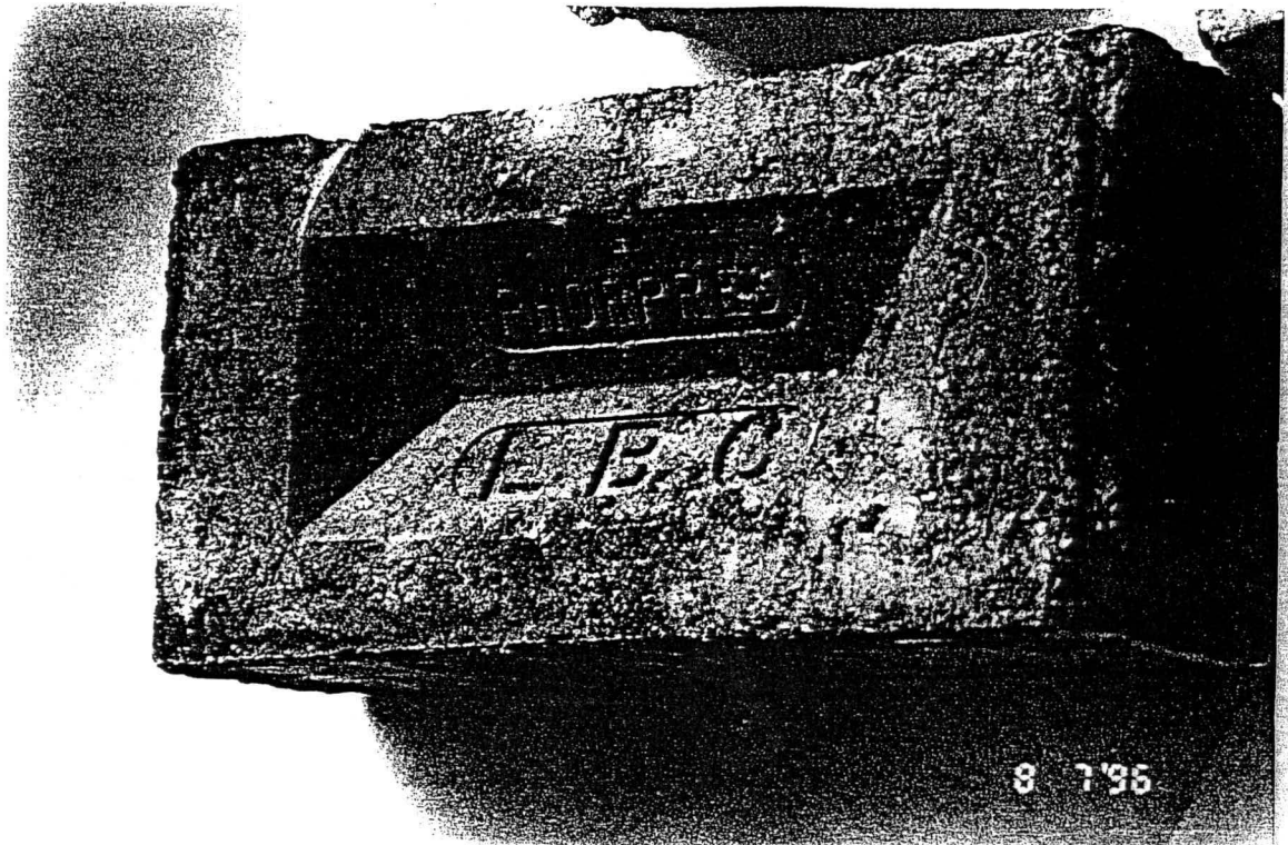
Fig. 4 Frog of yellow Fletton brick from Cork Street, London, from building dated 1910.
