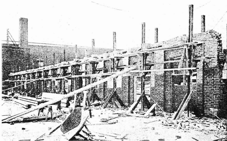
FIG. 1. The Gilbreth scaffolding in use.
