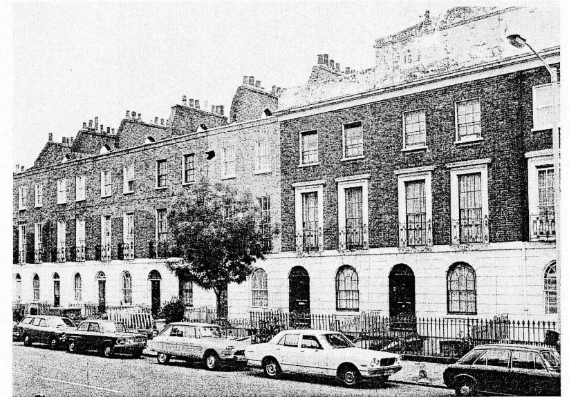
Fig. 1: The flat frontages of speculative London: Liverpool Road, Islington, 1834.
