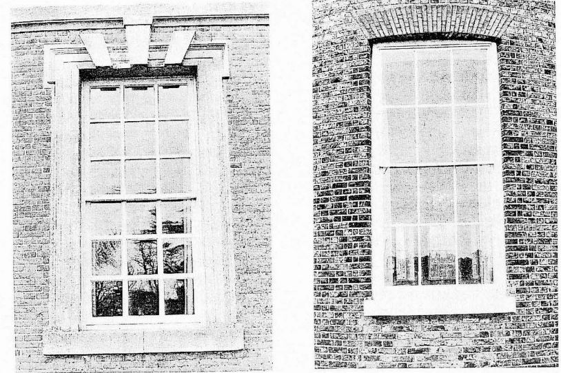
Fig.2 Raynham Hall, Norfolk: The Garden Front. Window to old State Bedroom c1703 showing typical reflection in crown glass of the period. Pane size: 12 3/4" x 15".
