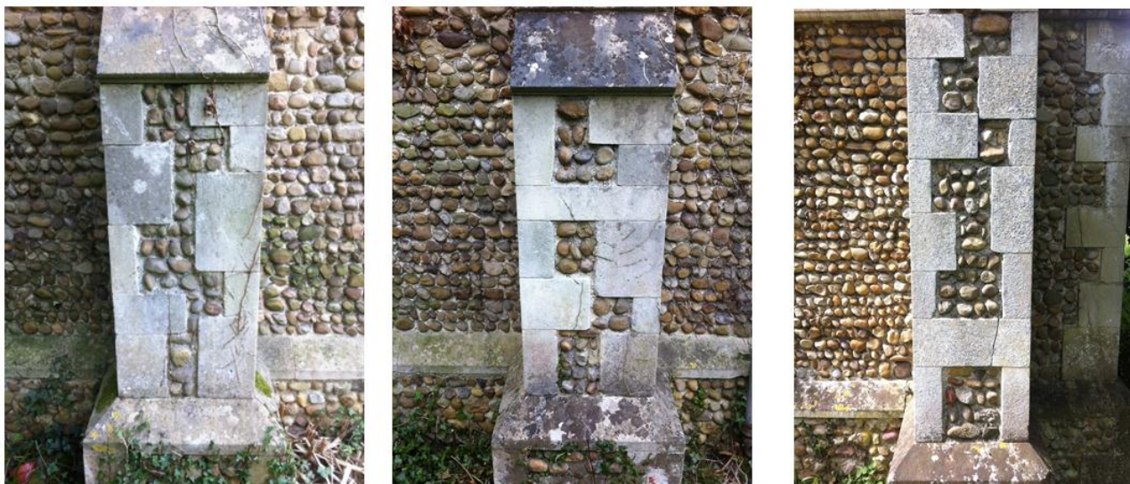
Plate 7: Comparison of stone dressings on buttresses
