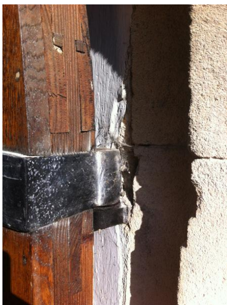
Plate 8: West Door showing red pine overlaid with oak slats hung on iron hinges
