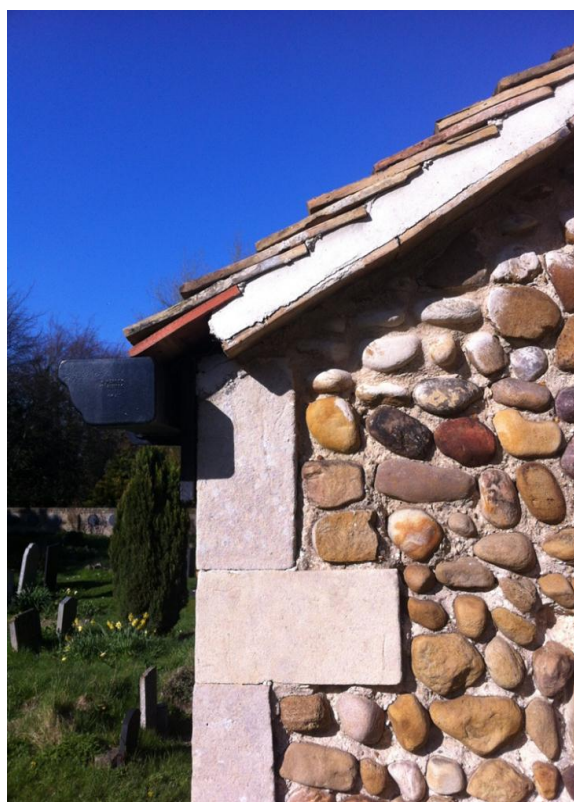
Plate 9: Projection of vestry showing coursing of flint, alternating Ketton and Clipsham Limestone dressing and clay tiles
