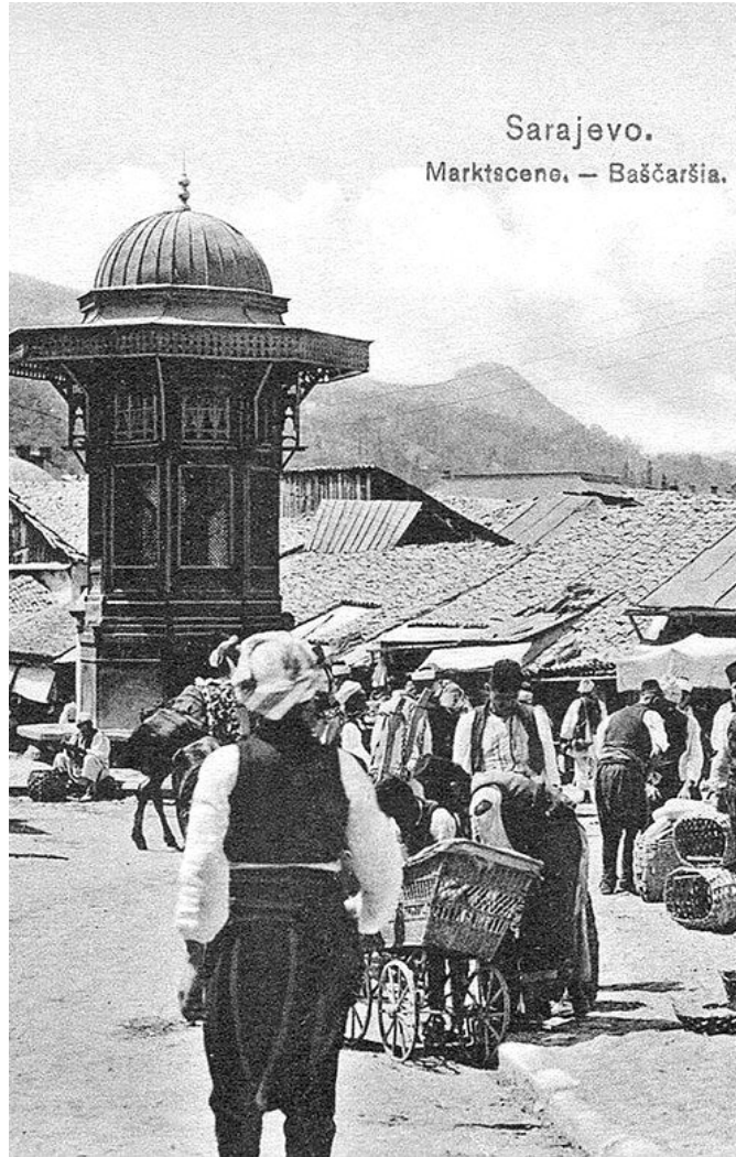
Fig 3.6 The Sebilj of Sarajevo's central Baščaršija market. Ottoman identity is expressed through ornate Islamic wooden panels and canopy details, and the form of the raised limestone platform and domed copper roof.
