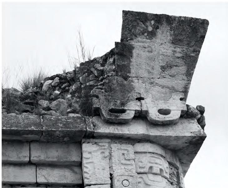
Figure 9: Cornice of the South Façade on the PG, with five specialised constructive pieces. Photo: Riccardo Montuori, 2018
