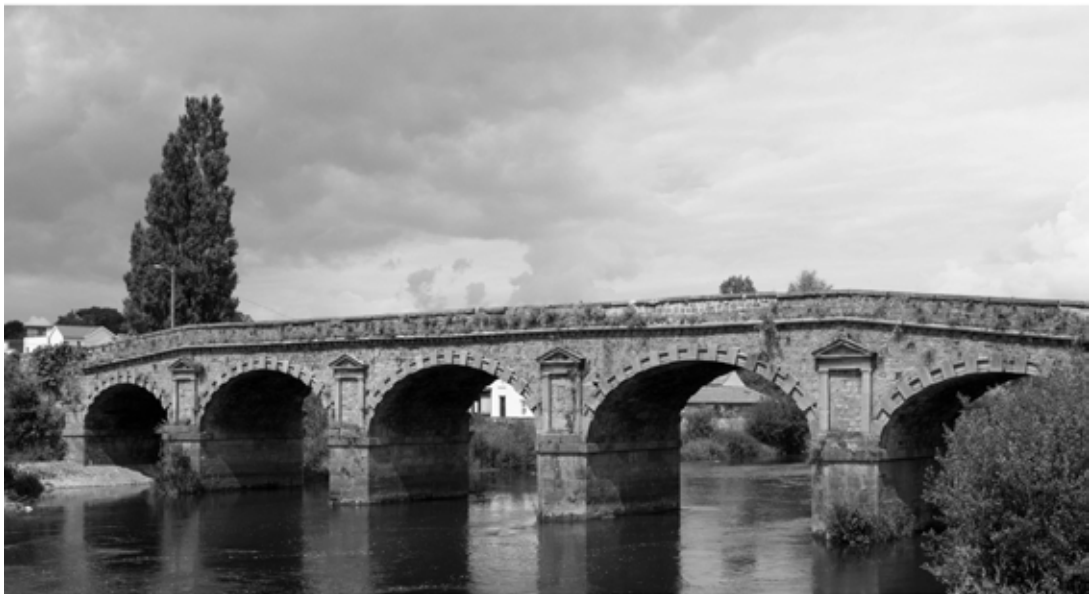
Figure 6: Green's Bridge designed by George Smith and constructed by William Colles.
