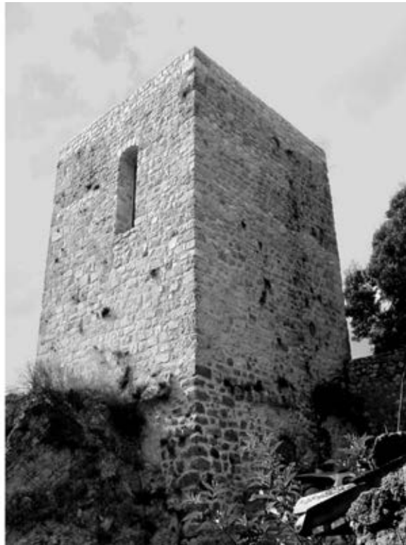
Figure 4: Square tower of Civita d'Antino.
