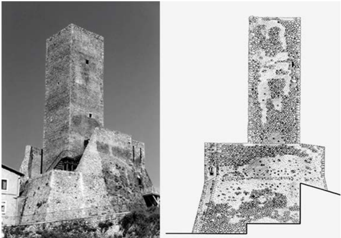
Figure 3: Introdacqua tower. On the left view of the south-west front; on the right drawing of the northern elevation. [Lab. of History, Department of Architecture, Unich]
