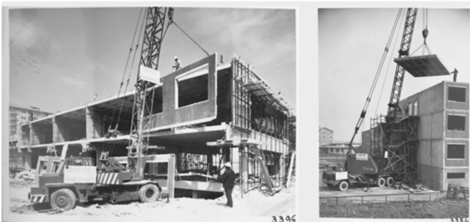
*Figure 7: Schools built using heavy prefabrication systems in Milan. Source: ACS-SGI, folder 4091-265, Edilizia civile 2*
