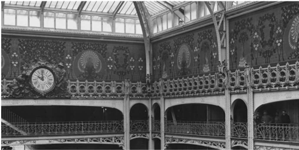
Figure 2. Magasin 2 La Samaritaine, Paris. Architect, Frantz Jourdain. Construction of main atrium using steel framing, c. 1905-10. Unknown photographer, La Samaritaine Archives.
