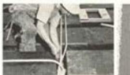
Placing electrical conduits in a bridging joint. All conduits are thus placed, eliminating necessity of extra space for service ducts.
