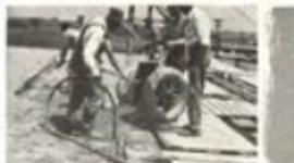
Concrete is being poured here over the steelforms and around the reinforcing steel. The final step is removal of steelforms and lumber after concrete sets.
