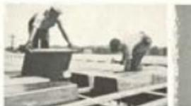
Erring steelforms on open wood covering preparatory to placing reinforcing steel. Use of steelforms means a saving in lumber.
