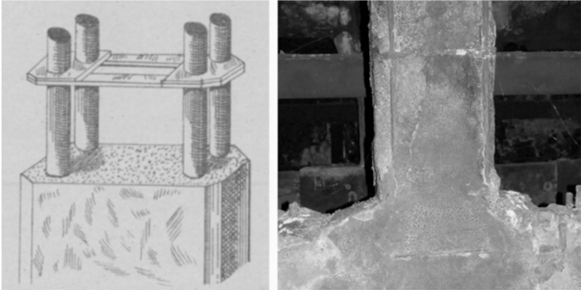
Figure 10: Reinforcement details of a column according to Ritter (left) and as built (right). Scan (left): from Hennebique company magazine *Le Béton Armé*, Jul.1899, p. 13; Photo (right): Kuban 2020.
