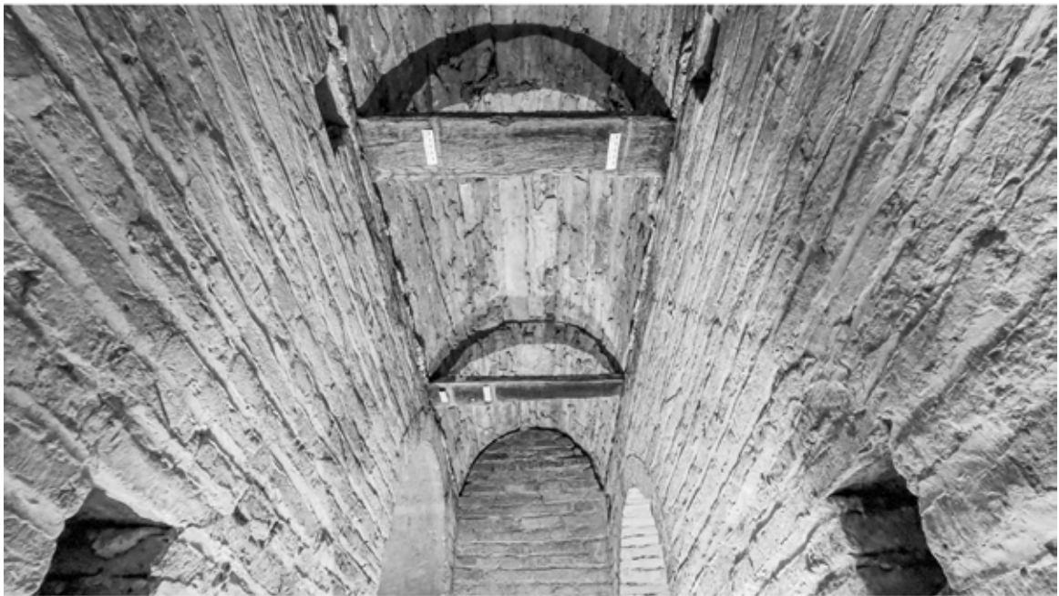
Figure 2: Boards used for vaulting the corridors of the front façade in the thirteenth century (picture: author)
