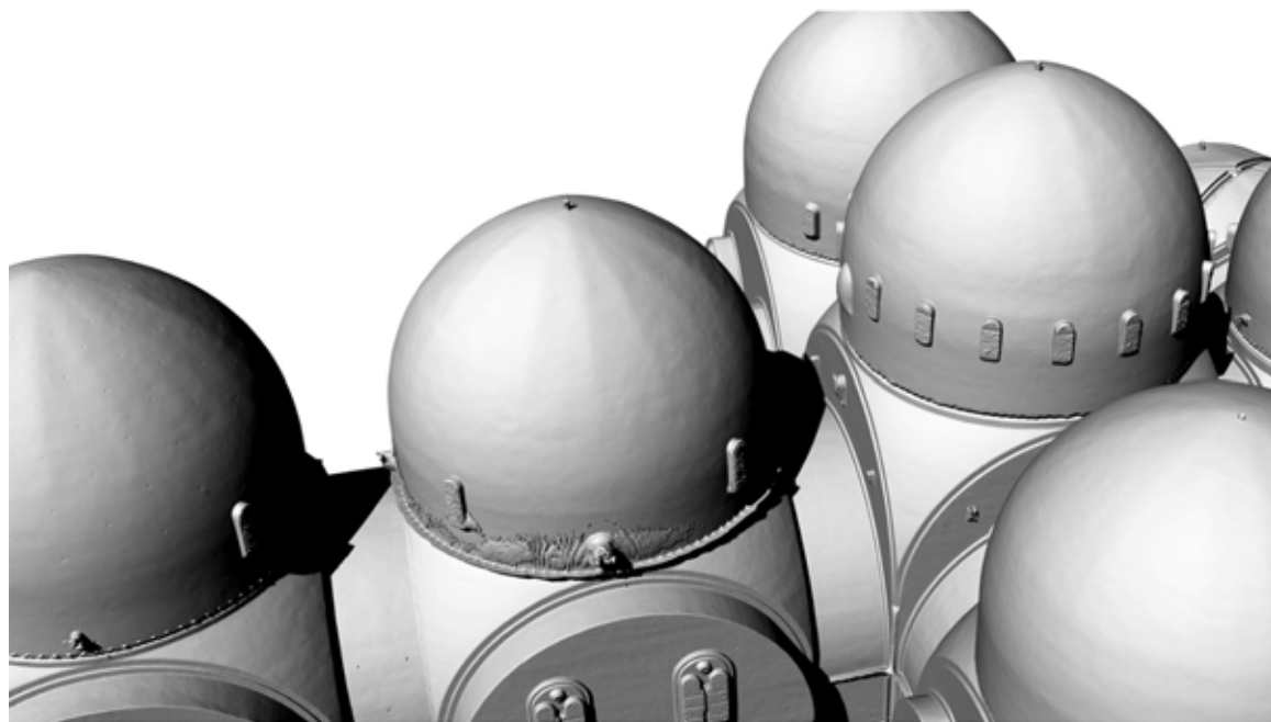
Figure 7: The meshed model of the intrados of the domes reveals traces of centring (model: author)
