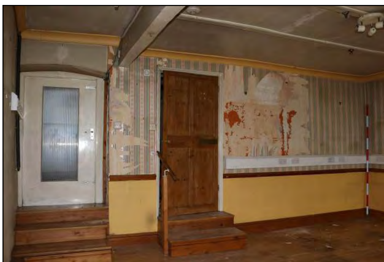
Plate 16 Room GF01 (Range 1) with modern doors and dry-lining, taken from the south (DP101)
