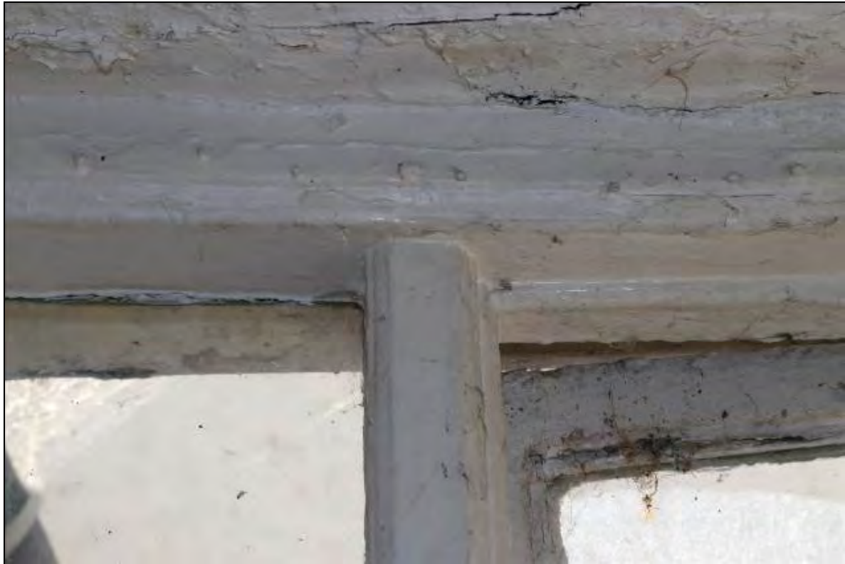
Plate 21 Detail of the moulded mullion on the 18 th century three-light casement in GF02 (Range 2) (DP76)
