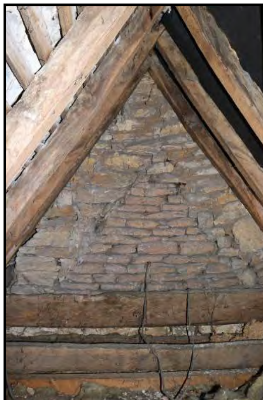
Plate 40 Roof structure (Range 3) showing north gable of Range 2 having been built up with Range 3, taken from the north (DP224)
