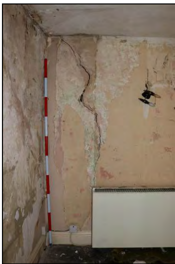
DP 135 Detail of the west wall of Room FF01 (Range 1) showing cracking in the original fabric, taken from the east
