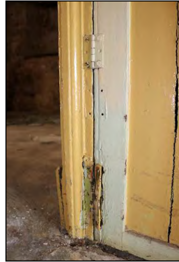
DP 92 Bottom of door below the staircase in Room GF02 (Range 2) showing H-hinge and impressions for lost hinges, taken from the west
