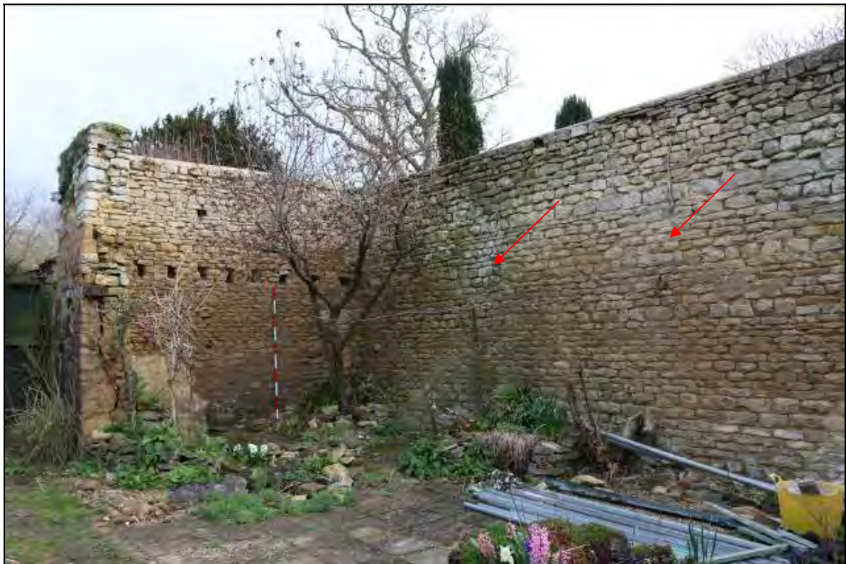
Plate 15 North and east walls of Range 6 showing blocked apertures for lost binding joists (indicated) and sockets for common joists to the left (DP231)
