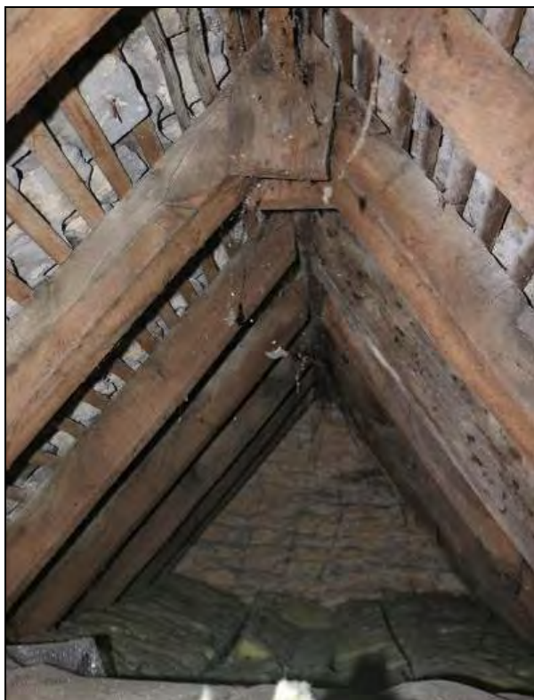
Plate 38 Roof structure over Range 1 showing rafter couples with occasional yoke piece, taken from the east (DP185)
