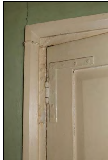
DP 142 H-L hinge on the 18 th century two-panel door at the south end of hallway FF03 (Range 2), taken from the north
