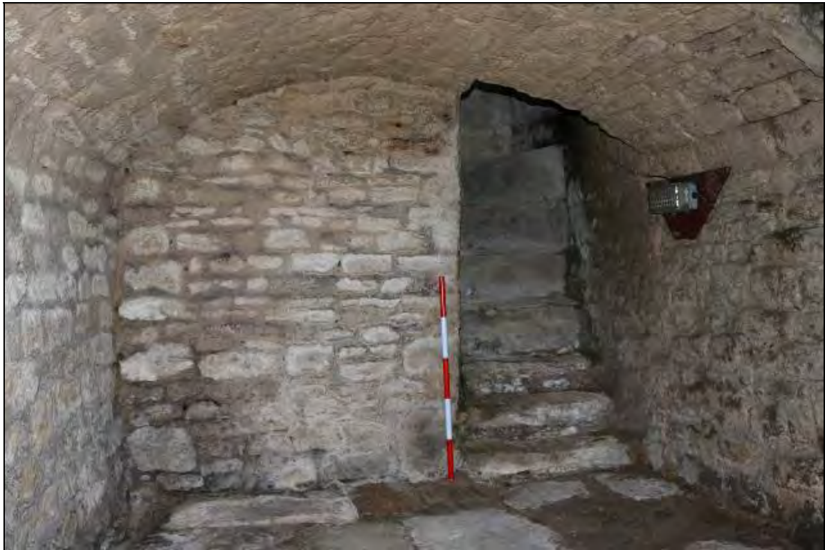
Plate 30 Interior of the barrel-vaulted cellar room CF01 (Range 3) (DP199)
