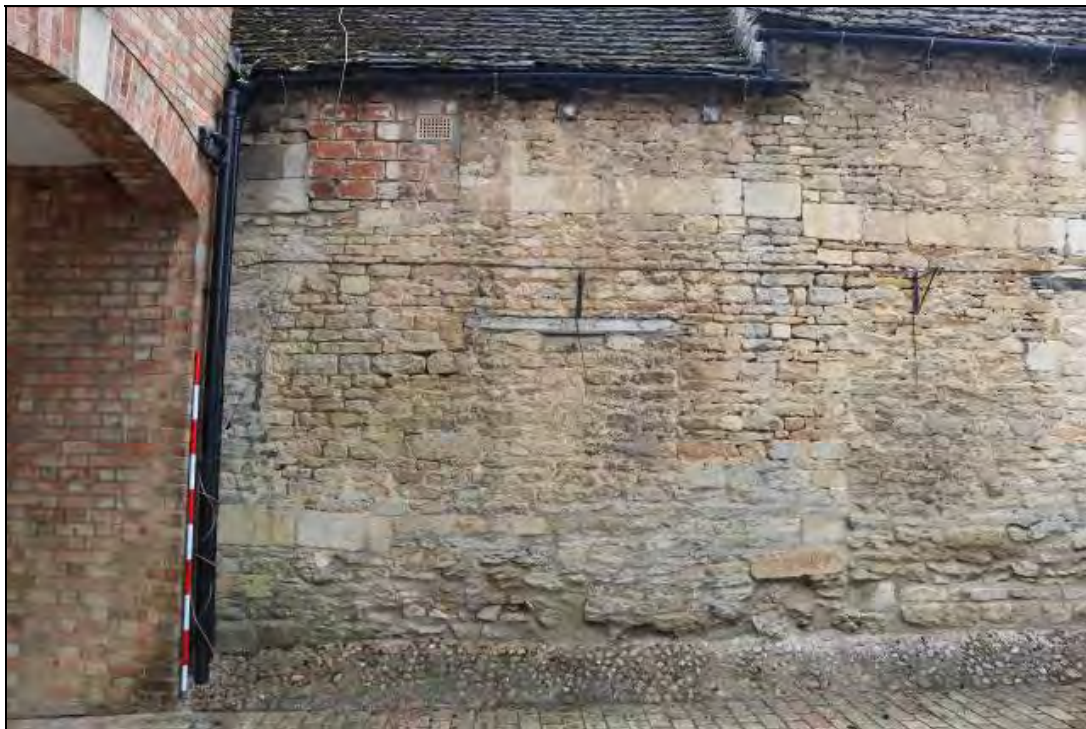
Plate 7 East side of Range 2 showing courses of good squared limestone with blocked apertures on both levels (DP240)
