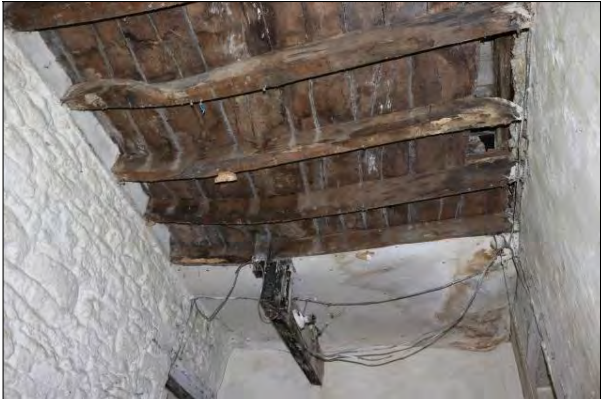
Plate 29 Ceiling of Room GF06 (Range 5) showing waney joists and additional truncated joist to the rear, taken from the west (DP54)
