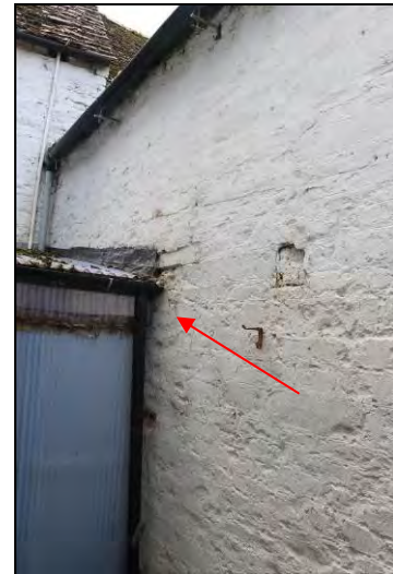
DP 22 External wall of the adjacent property to the west of the rear range showing blocked aperture (indicated), taken from the north-east
