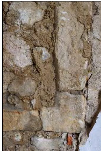
DP 106 Detail showing the chamfering of the stone frame on the window formerly lighting the staircase to the cellar (visible from within Range 4), taken from the north
