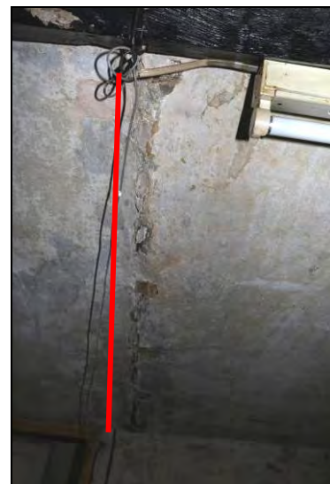
DP 72 Ceiling in Room GF02 (Range 2) showing remains of ephemeral partition (indicated), taken from the south
