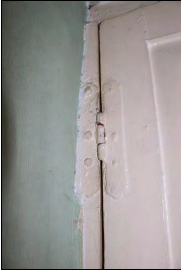
DP 139 H-hinge with shaped finials on the 18 th century door at the north end of hallway FF03 (Range 2), taken from the south
