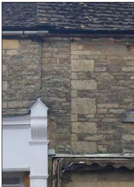
Plate 4 South elevation at first floor level showing depth of original west wall with 18 th century rebuilding to the right (Range 1, DP8)
