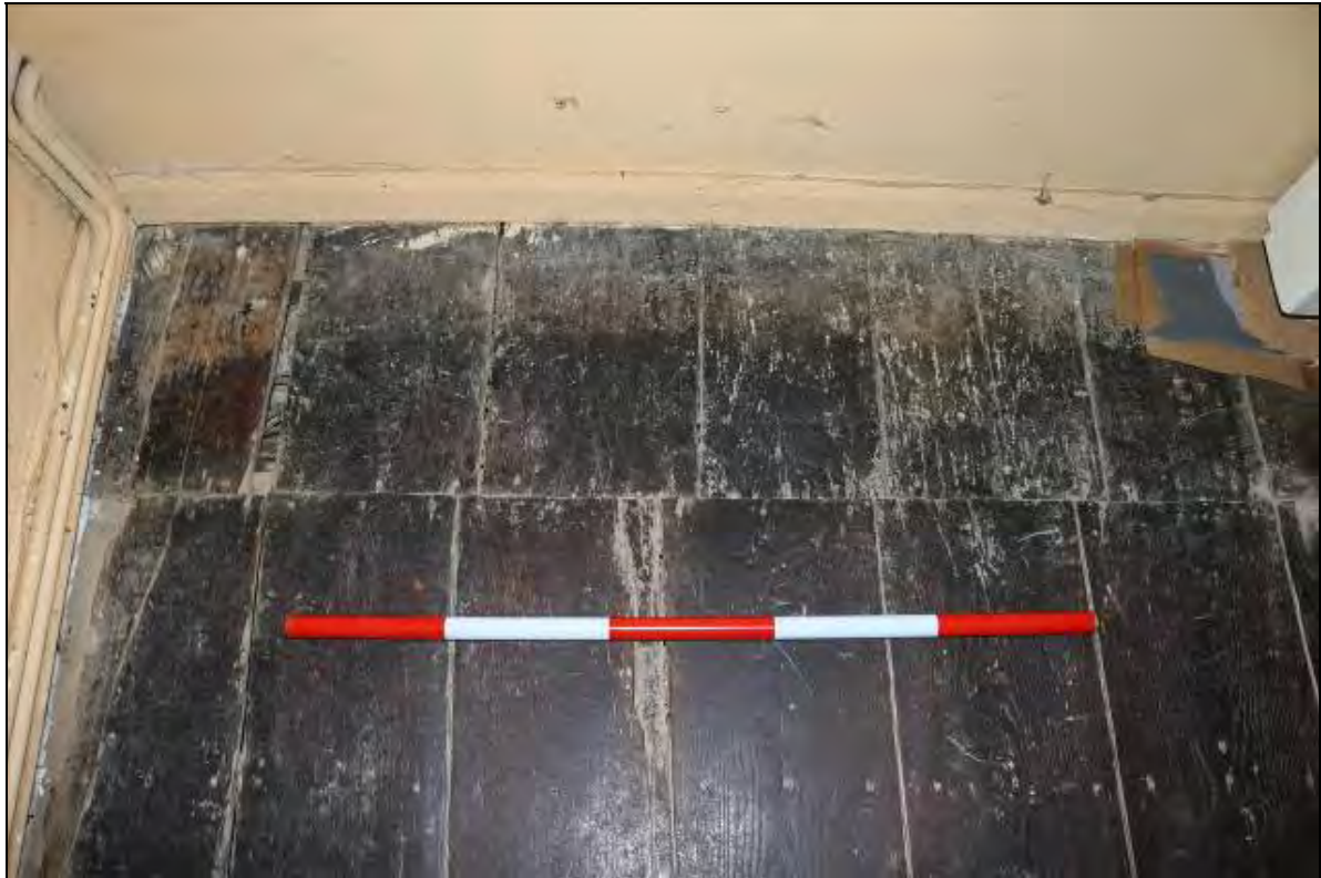
Plate 36 South side of the floor in Room FF05 (Range 3) showing straight joint between sections of wide historic floorboarding (DP154)
