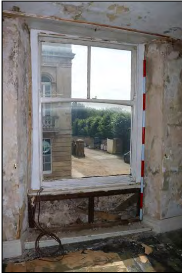
DP 133 Sash window on the south side of Room FF01 (Range 1) with 18 th century upper sash and late 19 th century lower sash, taken from the north
