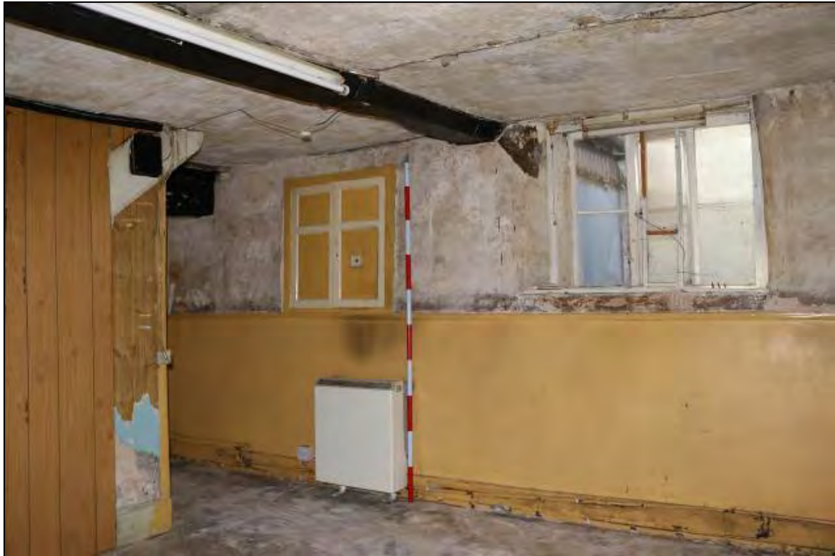
Plate 18 West wall of Room GF02 (Range 2) showing fabric including the late 16 th century binding joist and early 18 th century cupboard and window (DP83)
