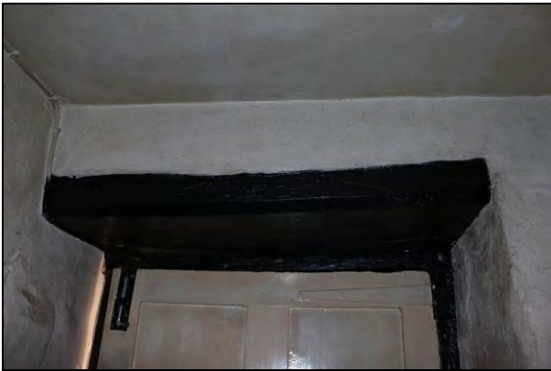
DP 67 South end of bridging joist in Room GF03 (Range 3) showing lambs tongue chamfer stops, taken from the south
