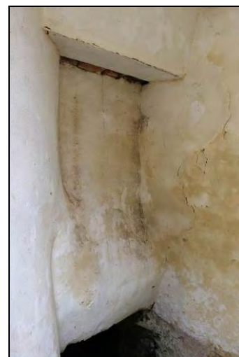
DP 108 Upper area of the staircase leading to the cellar (Range 3) showing position of blocked window aperture, taken from the south-west
