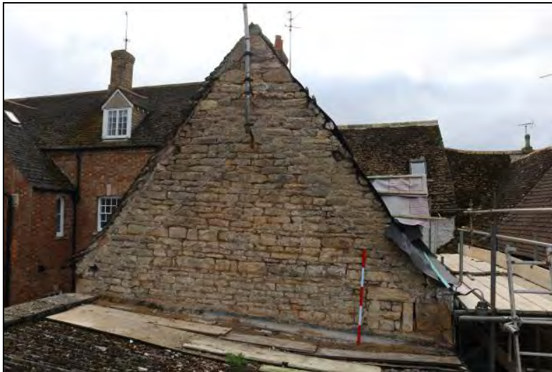
Plate 10 North elevation of Range 3 at upper level showing small blocked aperture to light former staircase and impression of lost roof pitch (DP234)
