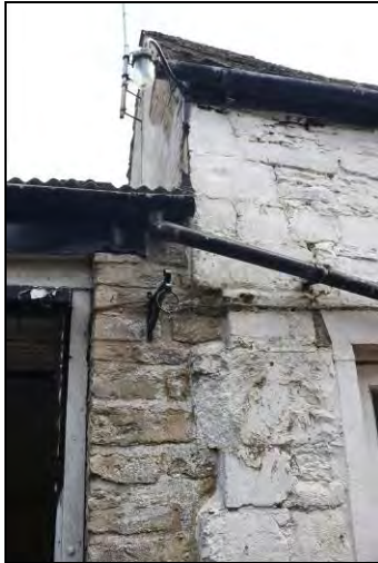
DP 19 Detail of the north end of the rear range (Range 3) showing quoining to the gable end, taken from the west
