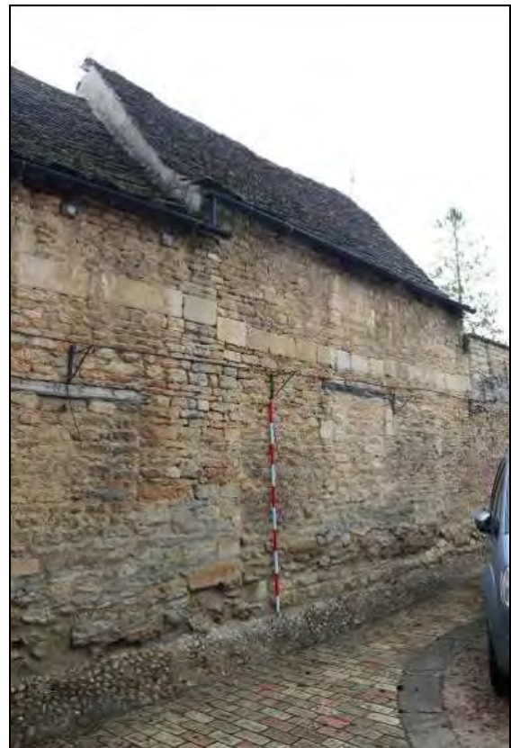
Plate 9 East side of Range 3 showing blocked apertures (DP242)
