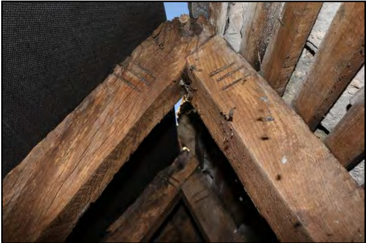
Plate 40 Roof structure (Range 3) showing rafter couples bridled at the apex with chiselled assembly marks (DP226)
