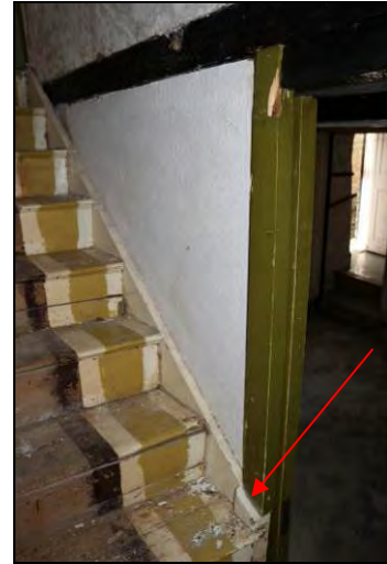
DP 122 Modern upper area of partition enclosing the staircase from Room GF02 (Range 2) with truncated newel below (indicated), taken from the south-east
