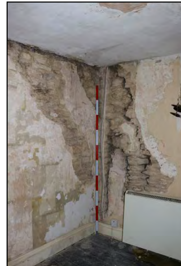
DP 214 South-west corner of Room FF01 (Range 1) showing structural cracking, taken from the north-east
