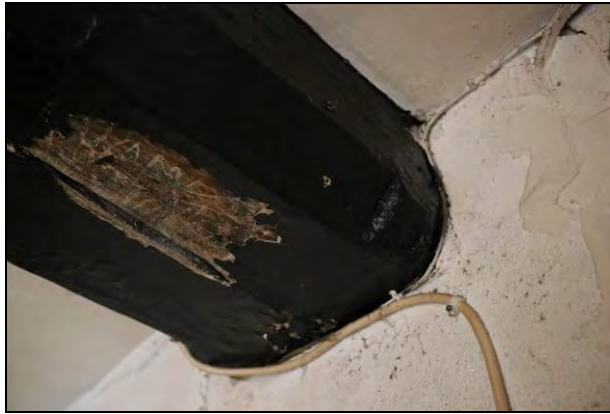
Plate 26 South end of bridging joist in Room GF03 (Range 3) showing lambs tongue chamfer stops (DP67)
