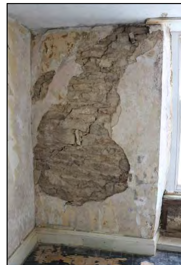
DP 216 Detail of the south wall of Room FF01 (Range 1) showing structural cracking, taken from the north
