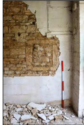
DP 104 Formerly external north wall of Range 3 (from within Range 4) showing stone framed window to light the staircase to the cellar, taken from the north
