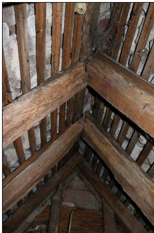
Plate 39 Apex of the roof structure over Room FF03 and FF04 (Range 2) showing bridled and pegged rafter couples (DP155)
