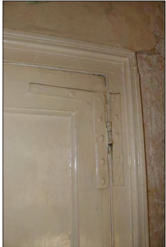
Plate 32 Detail of the H-L hinge on the 18 th century two-panel door on the north side of Room FF01 (Range 1) (DP127)
