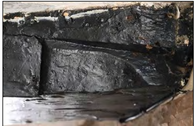
Plate 20 Large chamfer stop on the binding joist in Room GF02 (Range 2, DP99)
